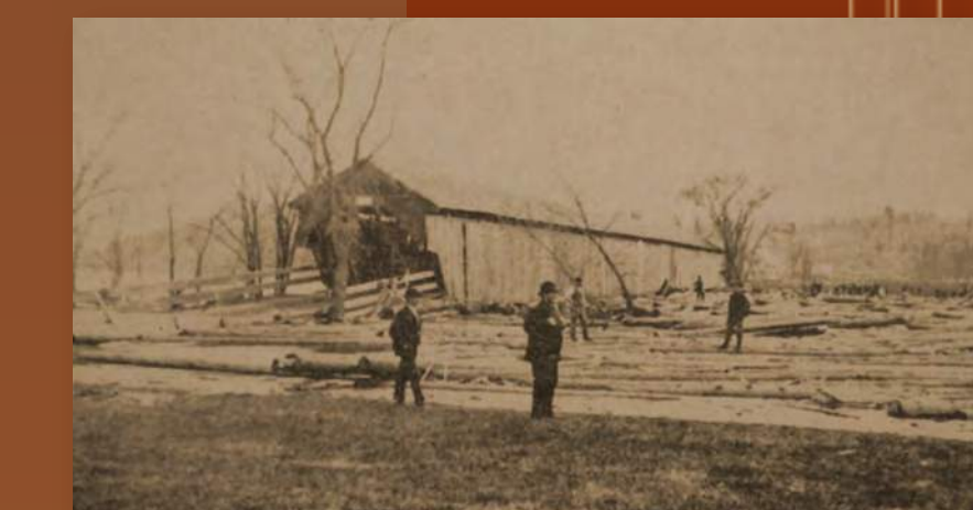
This 1890s view looking toward Vermont shows the second Lancaster- Guildhall bridge, built prior to 1844. It shows a log jam building up behind the bridge, caused by lumbermen floating logs downstream to sawmills, damaging the bridge in the process.
