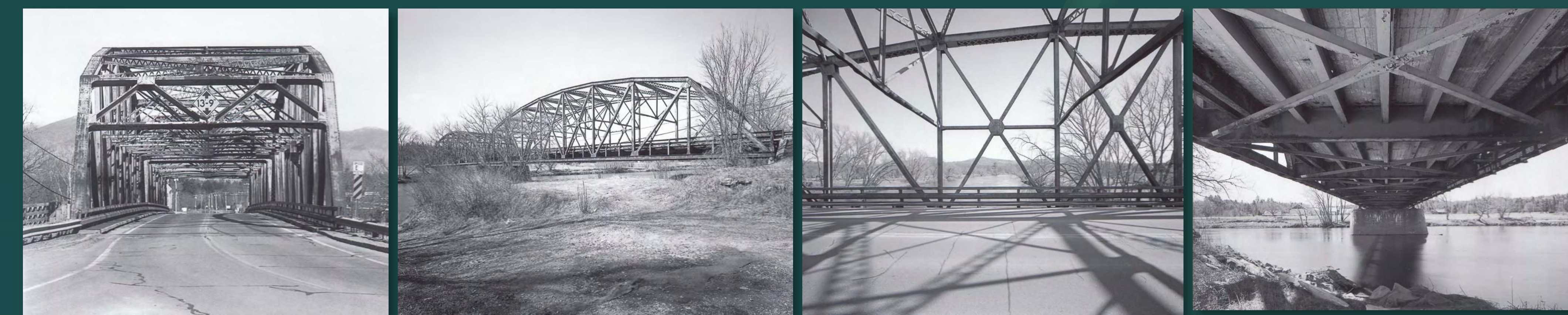
The fourth bridge of 1950, which was dedicated the Rogers' Rangers Bridge shortly after it opened, was a Parker high-truss bridge. It stood until being replaced in 2020. Views from left to right, (1) looking east from Vermont, (2) looking upstream at the eastern span on the New Hampshire side of the river, (3) detail of truss web, (4) view under bridge looking west toward Vermont. Image credit: Rob Tucher, photographer; HAER NH-56.
