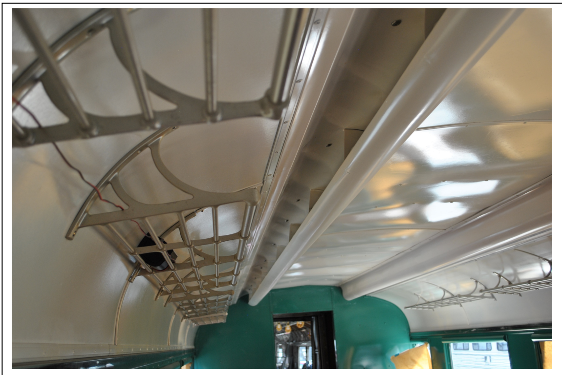
Photo 27. Car B, view of stylized light shade and baggage rack. View looking southeast toward rear (Patrick Harshbarger, photographer 7/20/23; HRI Neg. #23056 D1:040).
