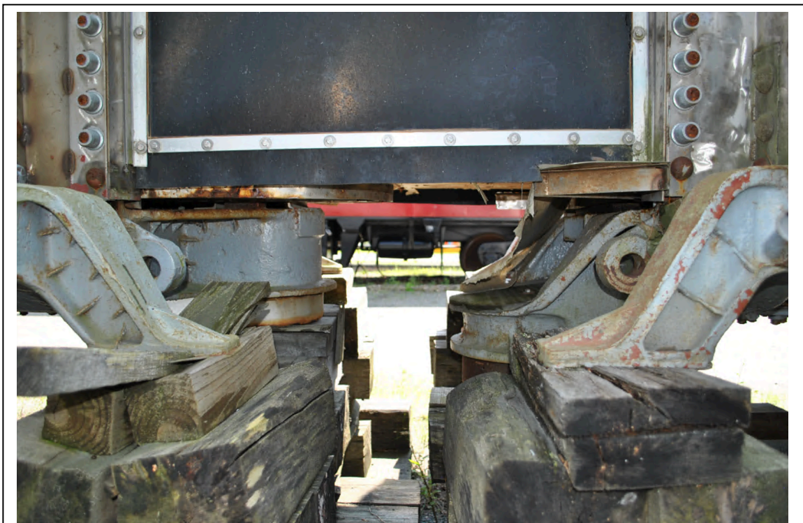
Photo 31. Detail of articulation between Cars A and B, looking southwest between the cars. The pivot casting is the large circular drum-like feature. The cars are currently disconnected (Patrick Harshbarger, photographer 7/20/23; HRI Neg. #23056 D1:087).
