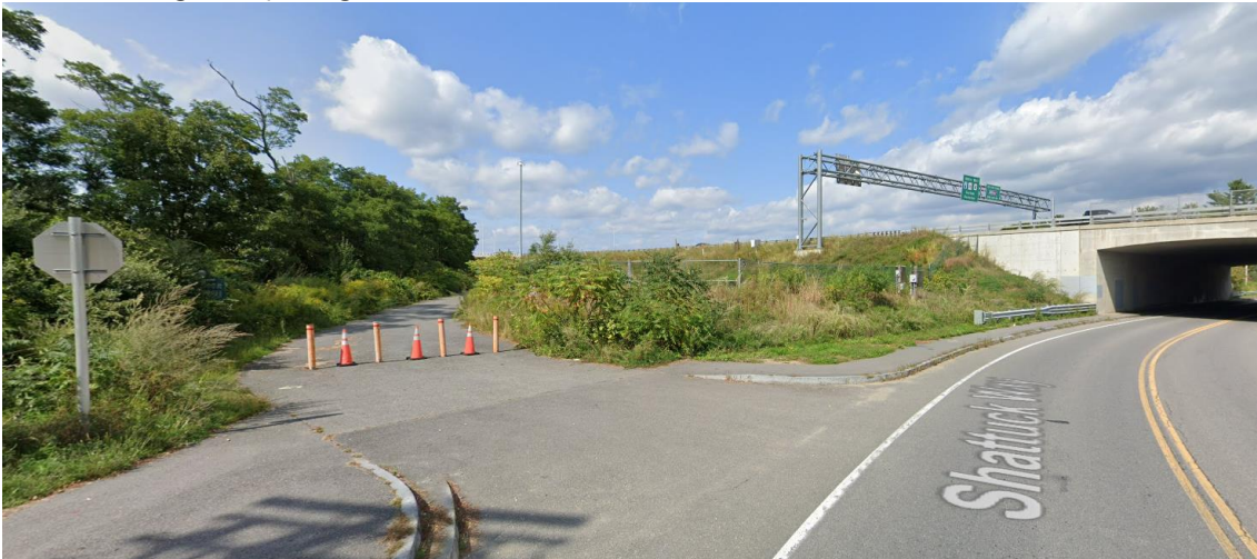
Photo 6: View from Shattuck Way of the beginning of the multi-use pathway leading to the GSB in Newington, showing the area within the 150-foot natural woodland buffer in the vicinity of the proposed water line conduit installation (Google Street View dated September 2019).
