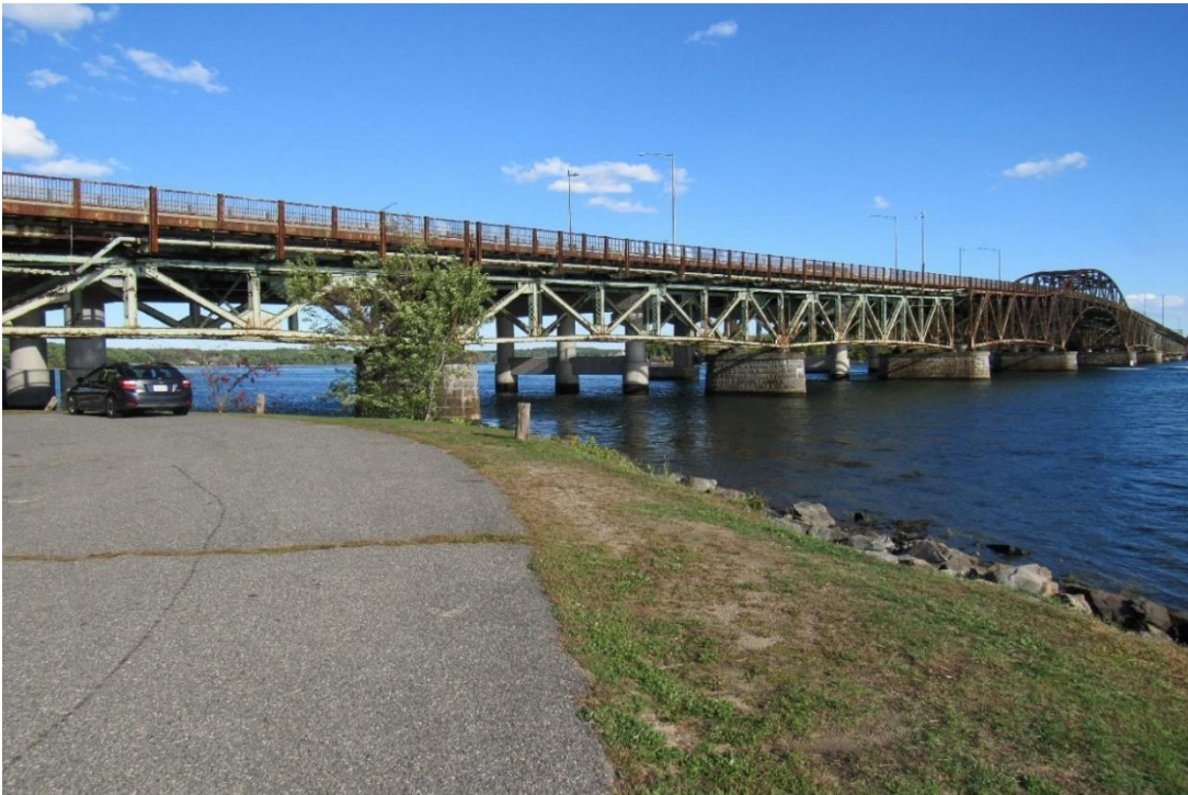
Photo 4: View east of General Sullivan Bridge from Hilton Park in Dover in the vicinity of one proposed temporary causeway, including the 50-foot waterfront buffer (9/27/2022).
