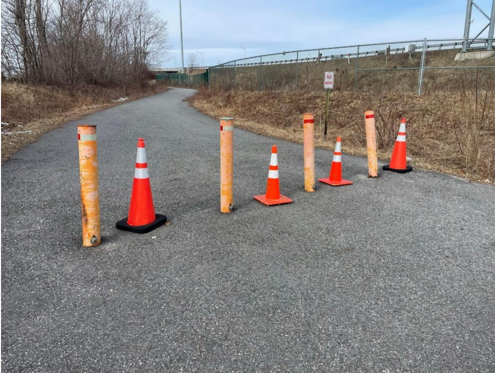
Photo 7: View of the beginning of the multi-use pathway leading to the GSB in Newington, showing the area within the 150-foot natural woodland buffer (2/5/2023).
