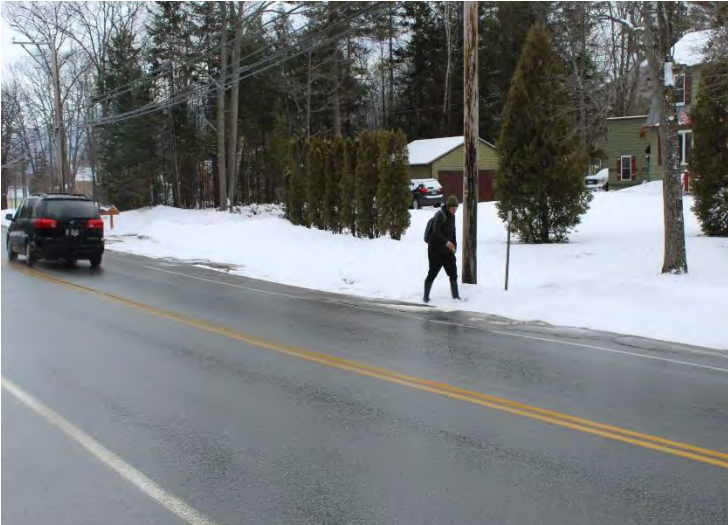
Area of proposed new sidewalk construction, approaching Multi-Modal Path
