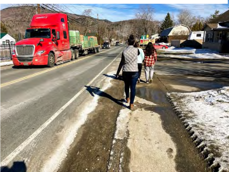
Existing sidewalk with no elevation
