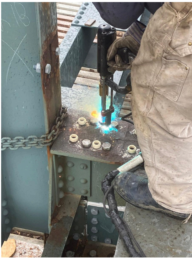
Shear studs being installed
