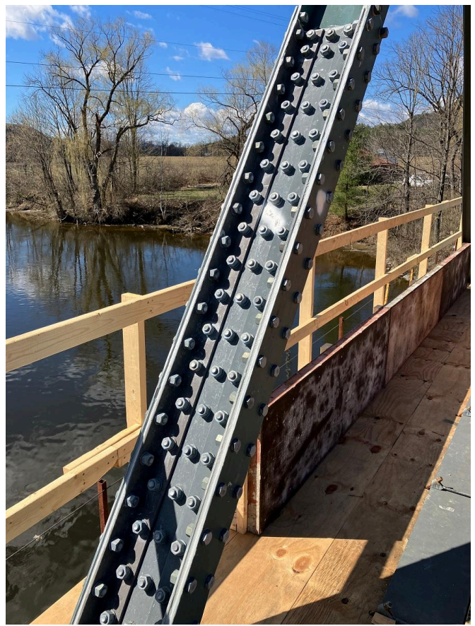
Repaired truss member
