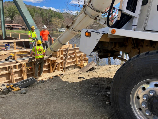
Replacing concrete at VT abutment
