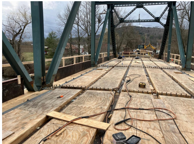
VT span with deck edge forms
