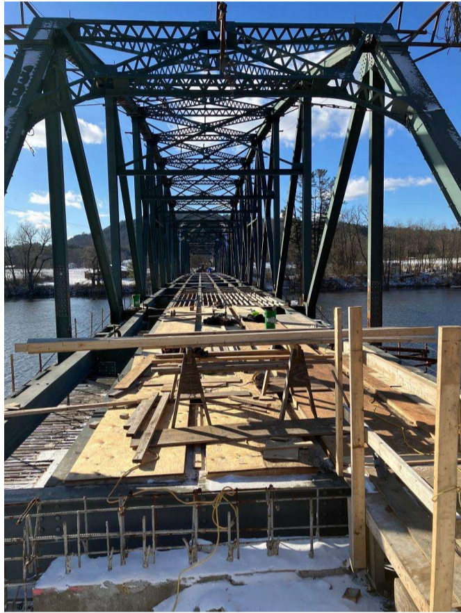
Deck formwork
