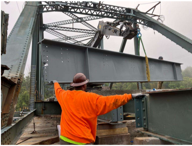
Setting of bridge floor beams
