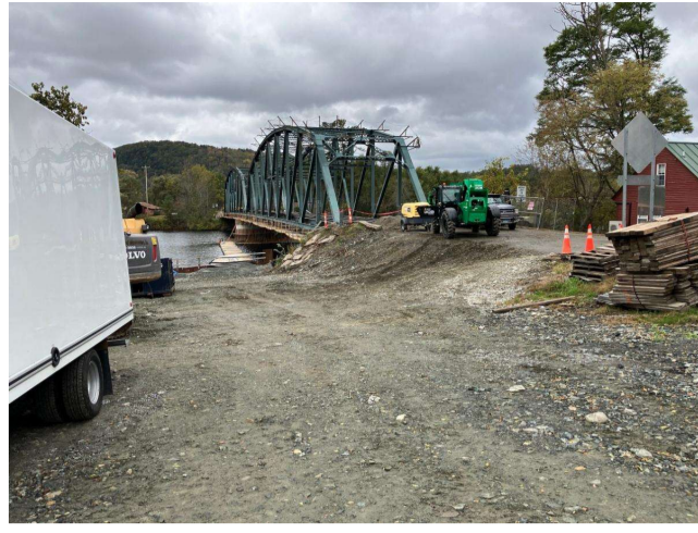
Cleaning at the bridge entrance after demolition activities
