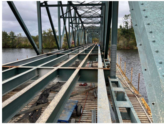
Structural steel repairs
