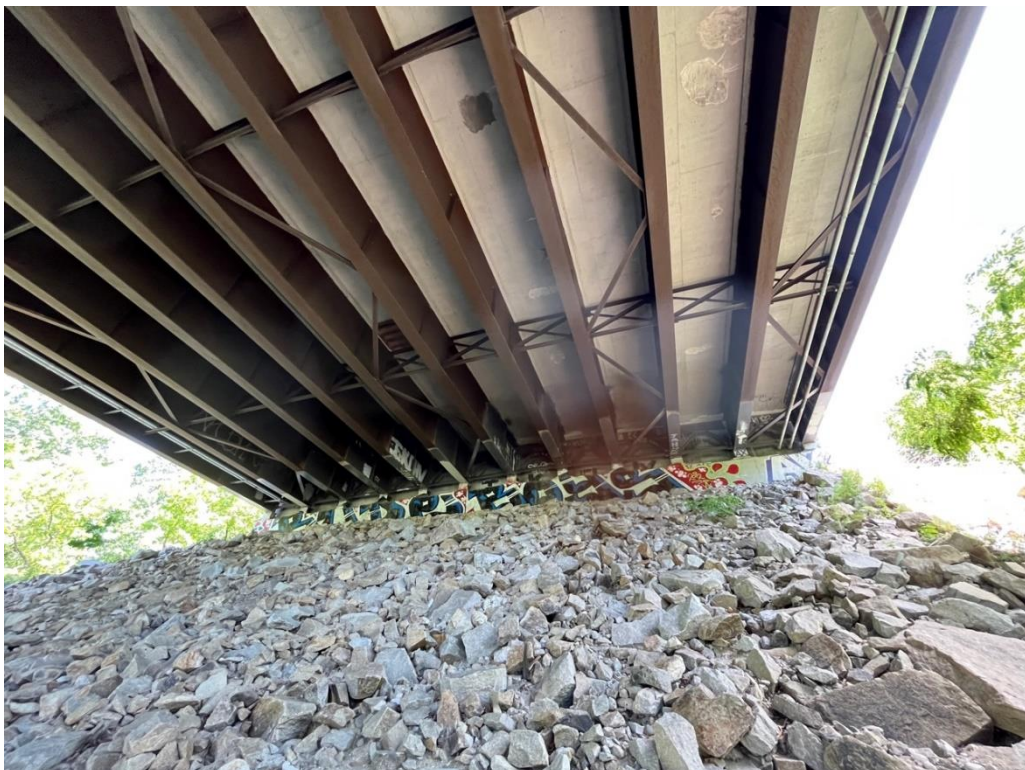
Photo 4. Looking east to bridge abutment at temporary impact area B (June 20, 2022)
