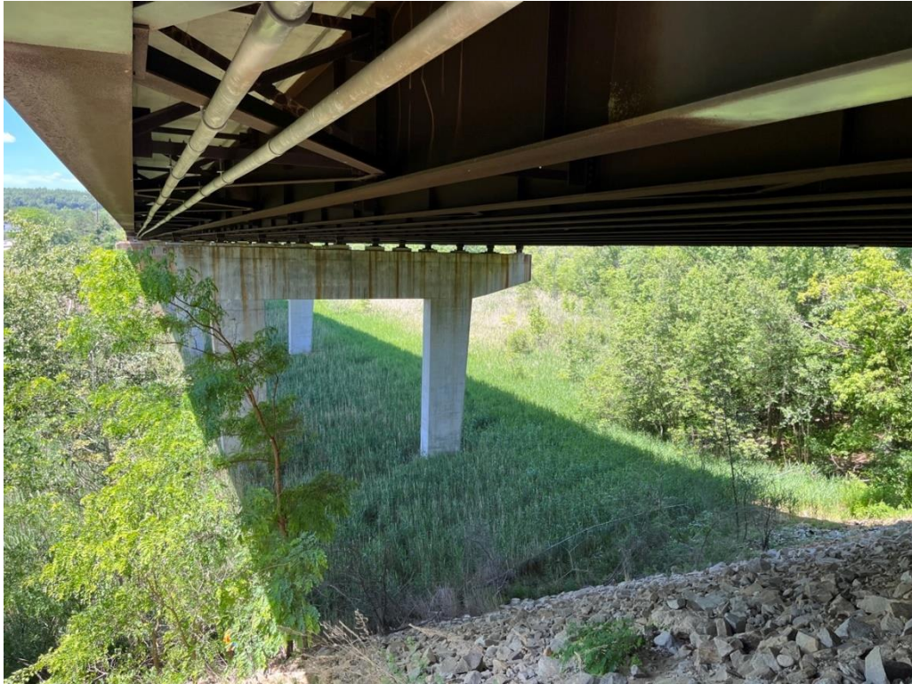
Photo 3. Looking west toward emergent wetland under temporary impact area B (June 20, 2022)
