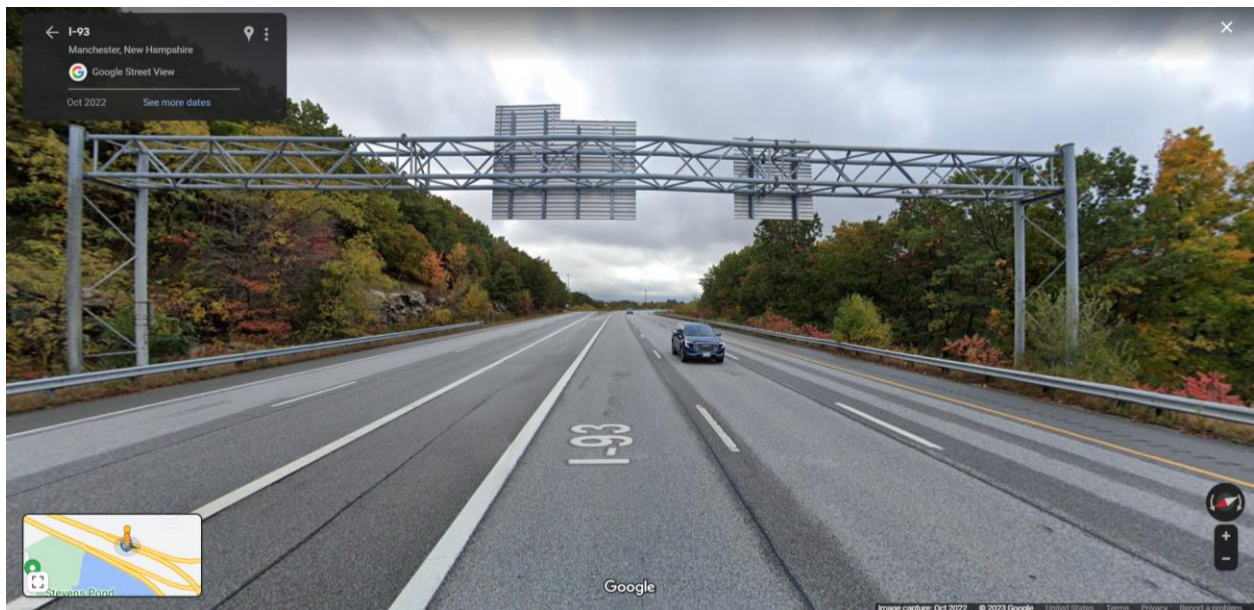
Photo 2. Looking east to temporary impact area A (Google Street View, October 2022)
