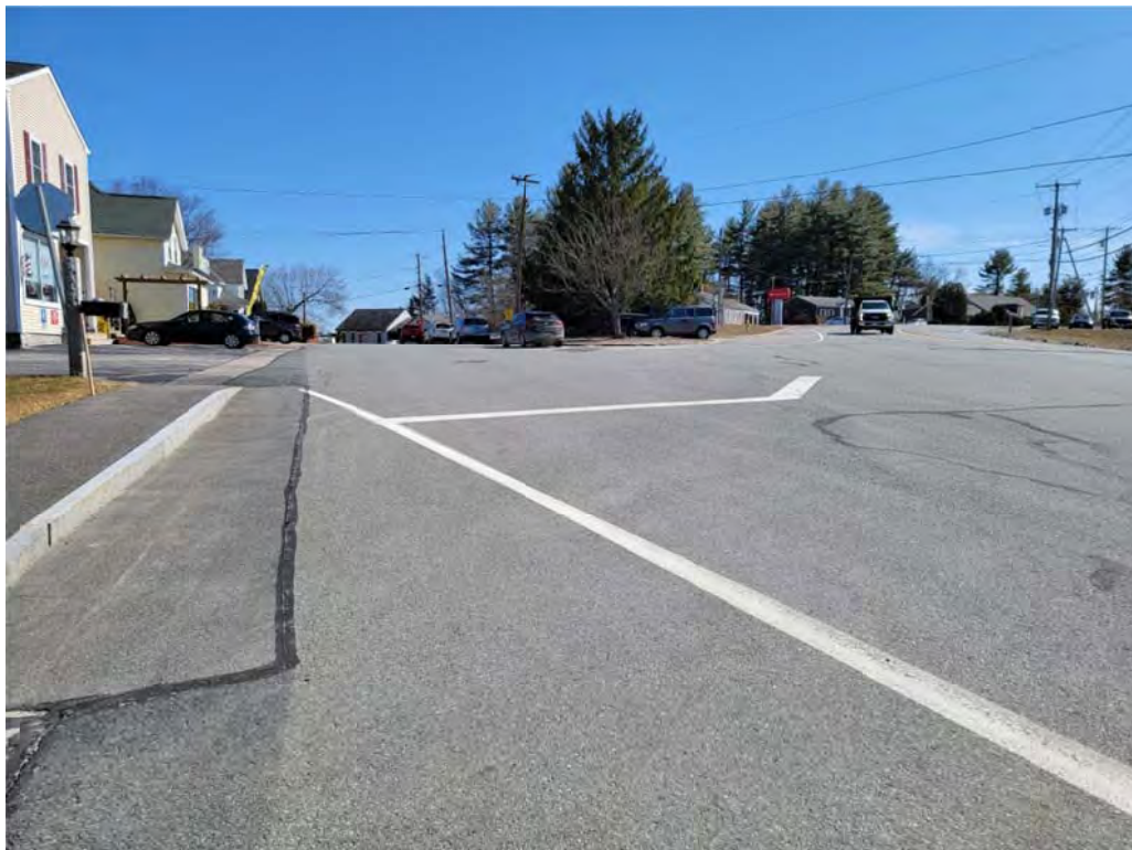
View of area where the sidewalk needs to cross over (3/19/2021)
