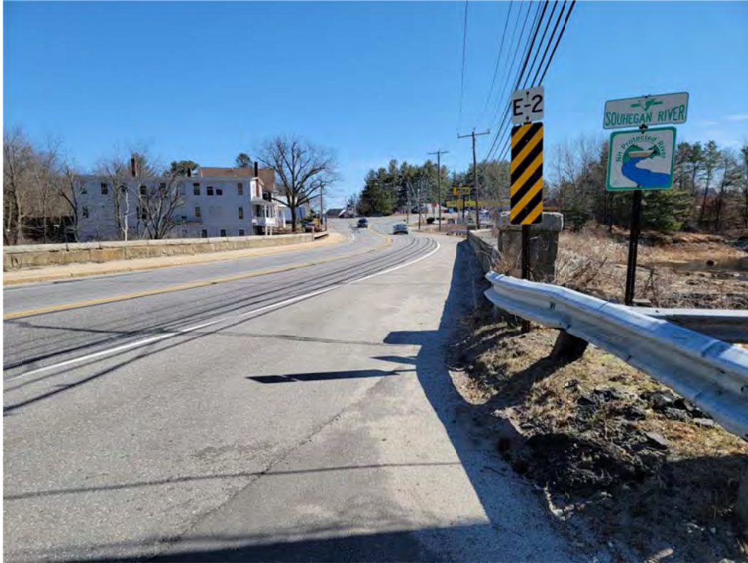
View southerly over Chamberlain Bridge sidewalk on east side (3/19/2021)
