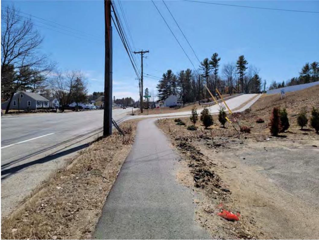
View southerly at East Chamberlain (new sidewalk up East Chamberlain (3/19/2021))
