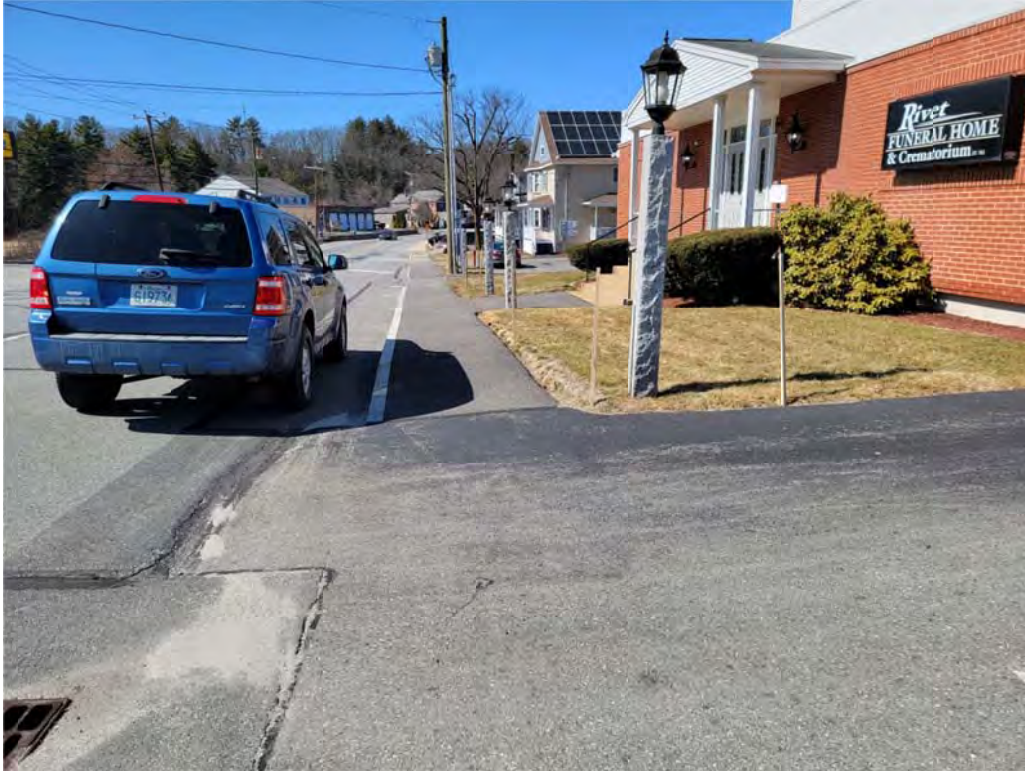
View northerly towards Chamberlain Bridge (sidewalk to tie into) (3/19/2021)
