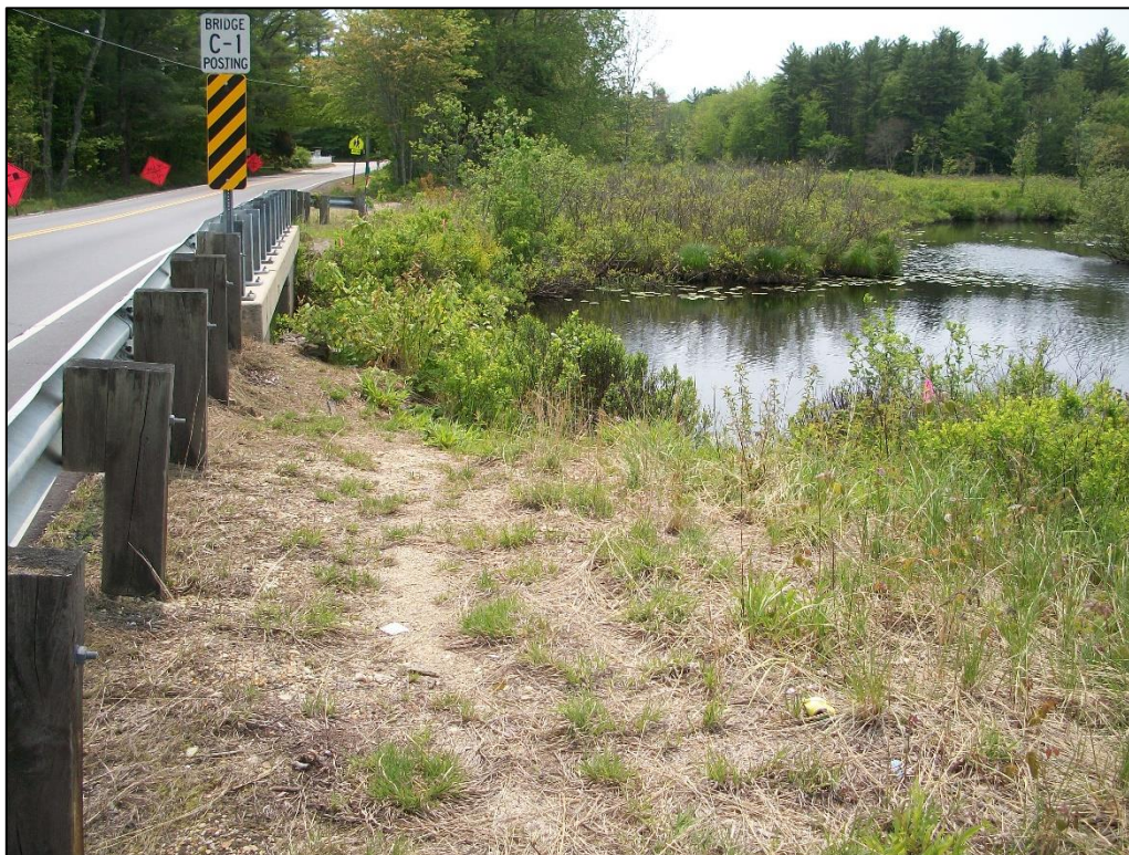
View south of Bridge No. 141/127
