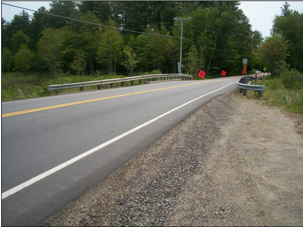
View southeast along NH Route 152 toward bridge
