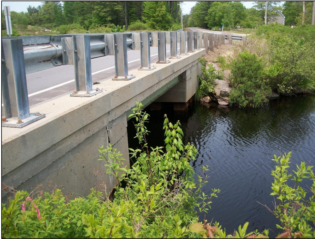
View northwest of Bridge No. 141/127 (NH Route 152 over North River)
