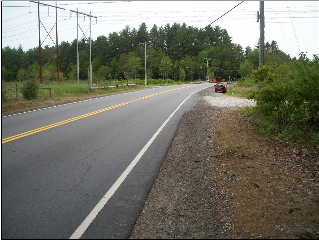
View south along NH Route 152 toward project area
