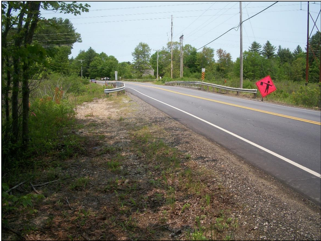
View north along NH Route 152 toward bridge
