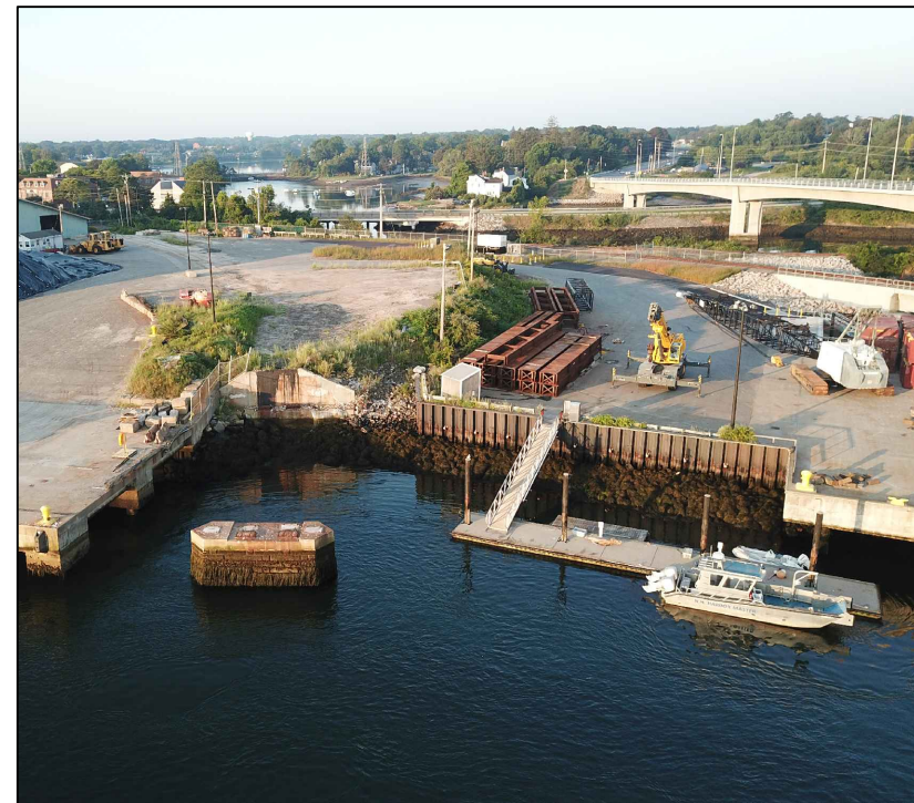
NORTH WHARF EXTENSION LOCATION LOOKING SOUTH
