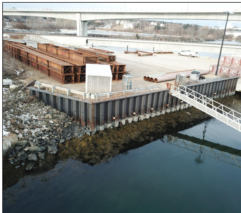
BARGE WHARF BULKHEAD LOOKING WEST (A1)
