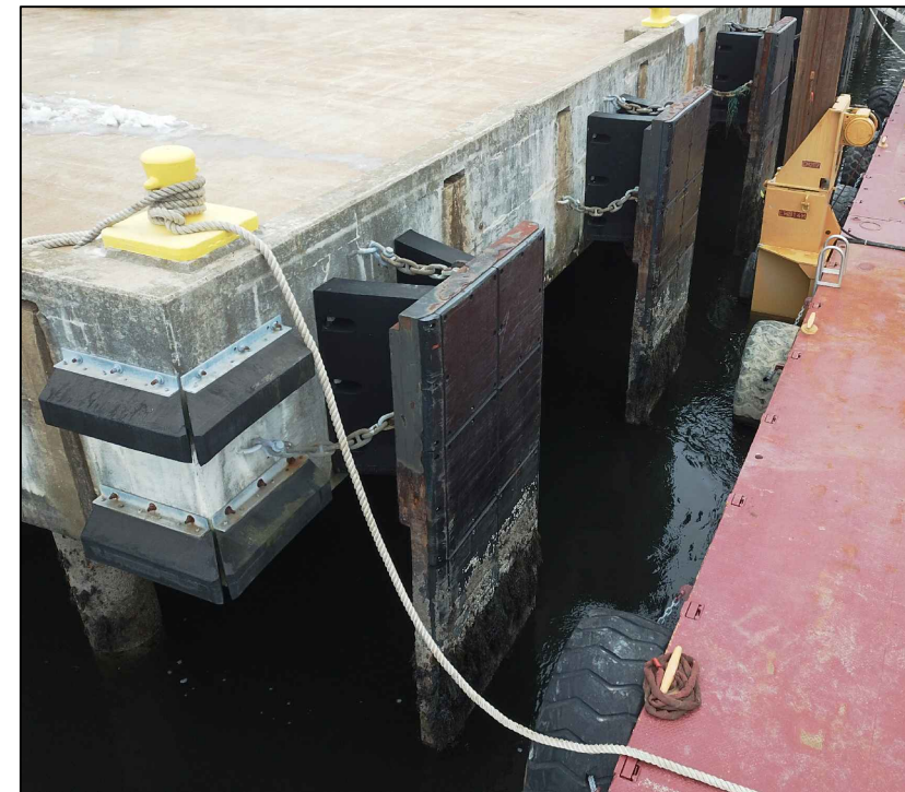
BARGE WHARF - FENDER SYSTEM LOOKING SOUTH
