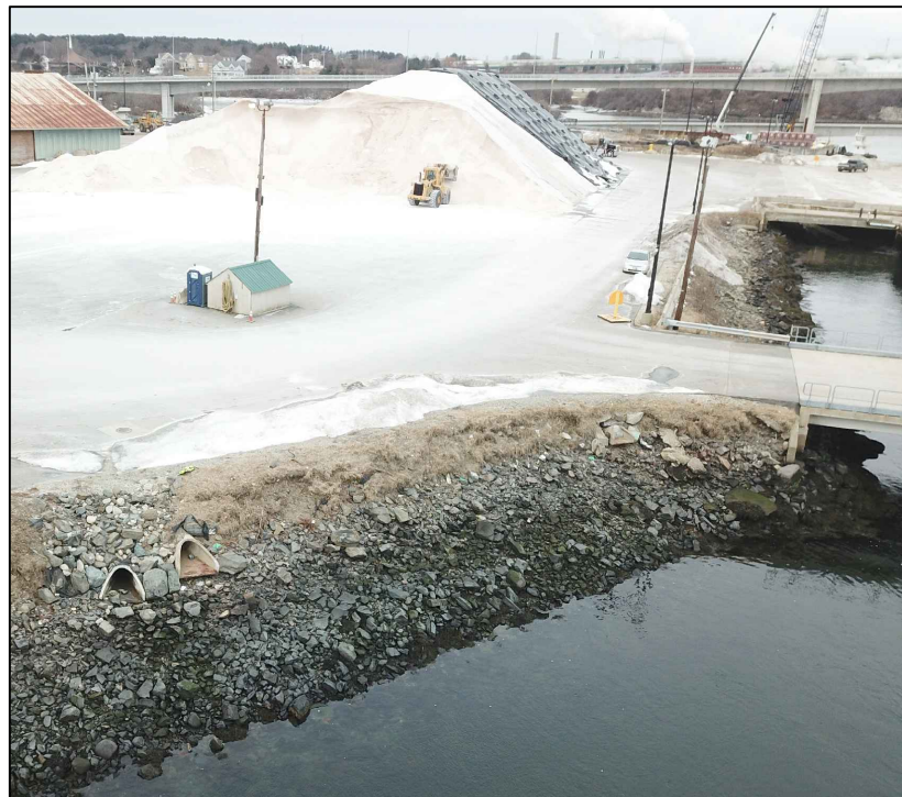
SOUTH WHARF EXTENSION REVETMENT LOOKING WEST
