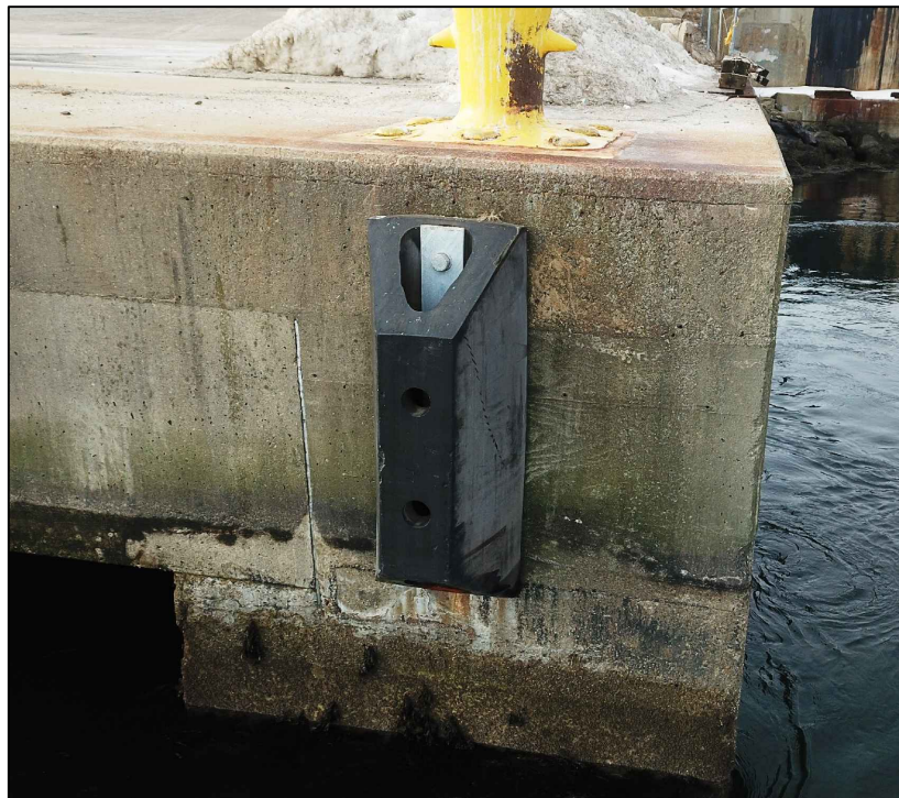
MAIN WHARF - FENDER SYSTEM LOOKING SOUTHWEST
