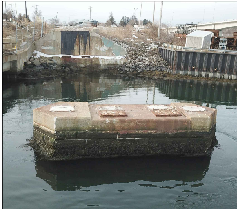
BRIDGE PIER 14 LOOKING SOUTHWEST (C3)
