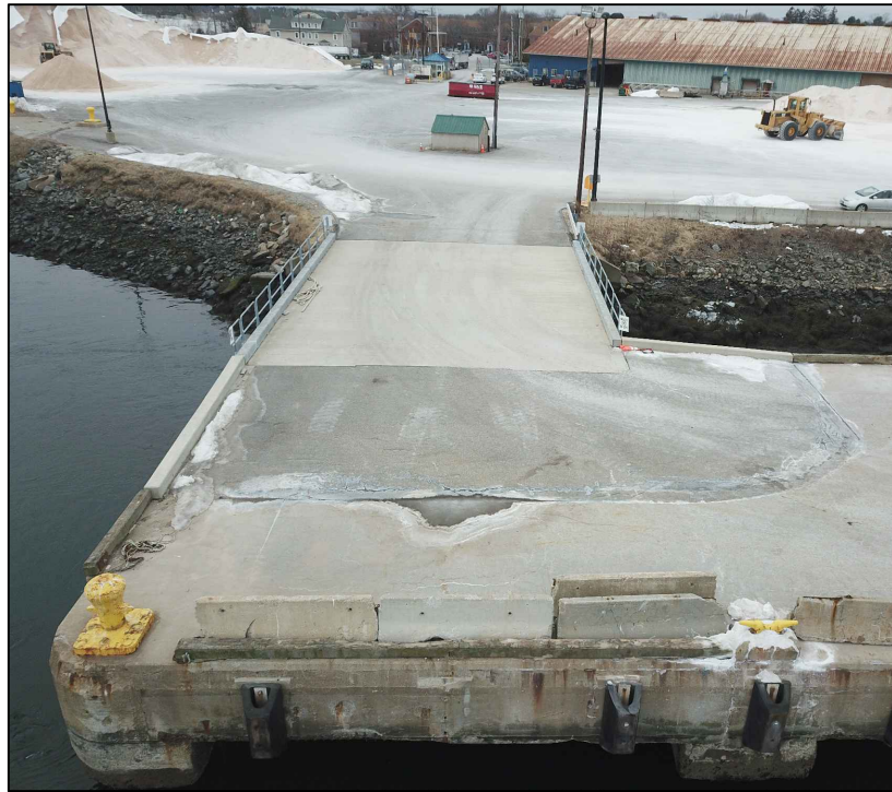
MAIN WHARF - SOUTH ACCESS BRIDGE LOOKING SOUTHWEST
