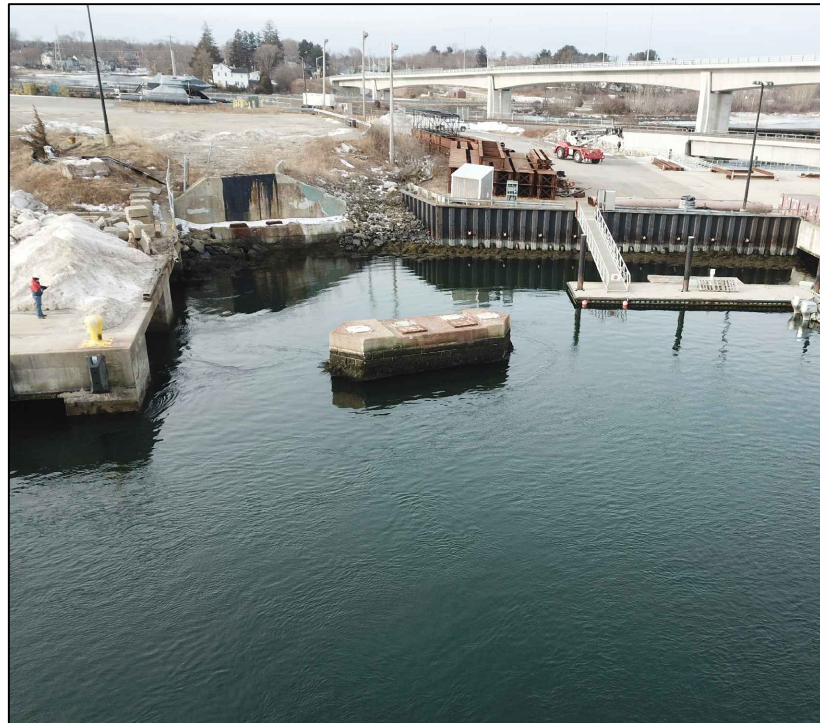
NORTH WHARF EXTENSION LOCATION LOOKING SOUTHWEST (C1)
