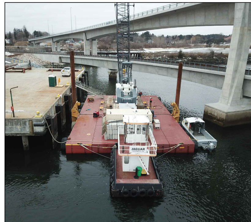
FLOATING DOCK - NEW LOCATION LOOKING SOUTHWEST (A4)
