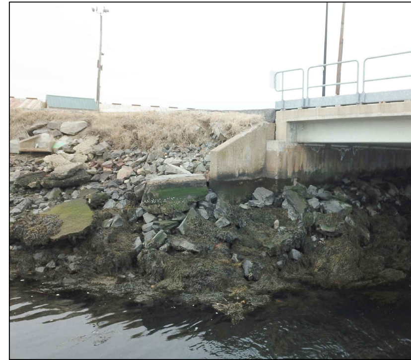
MAIN WHARF - BRIDGE ABUTMENT LOOKING WEST
