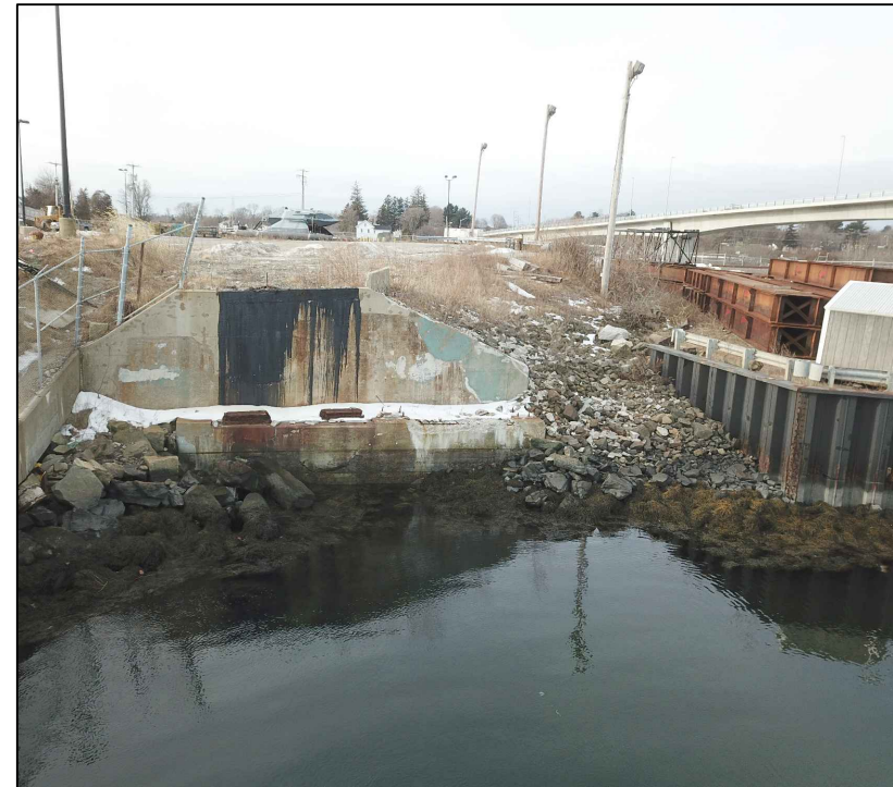
BRIDGE ABUTMENT 13 LOOKING SOUTHWEST (C4)
