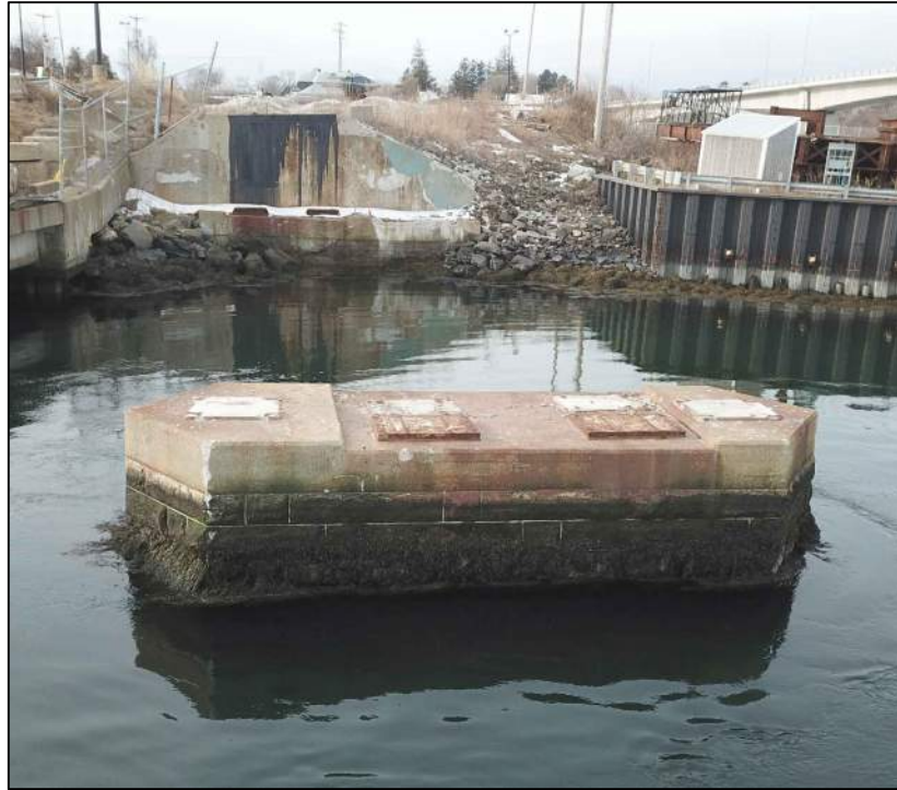
BRIDGE PIER 14 LOOKING SOUTHWEST (C3)
