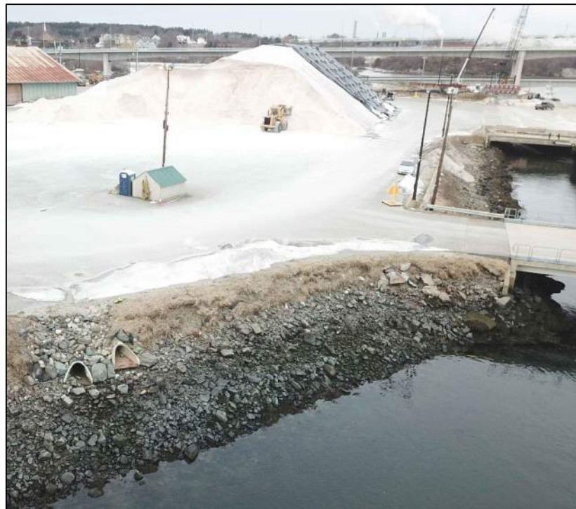
SOUTH WHARF EXTENSION REVETMENT LOOKING WEST
