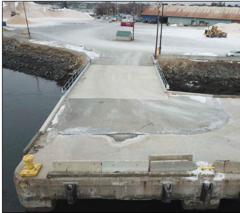
MAIN WHARF - SOUTH ACCESS BRIDGE LOOKING SOUTHWEST
