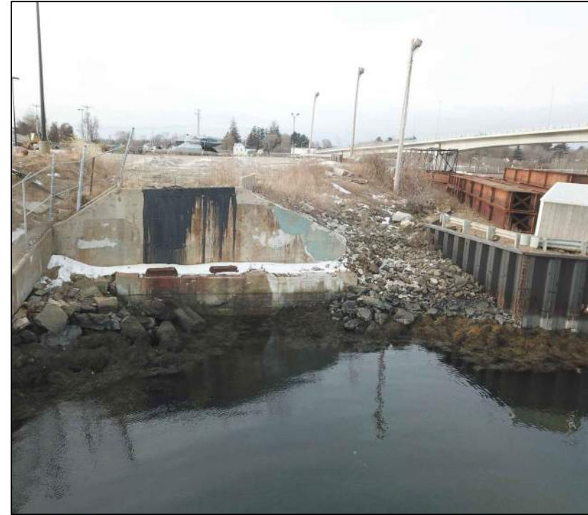
BRIDGE ABUTMENT 13 LOOKING SOUTHWEST (C4)
