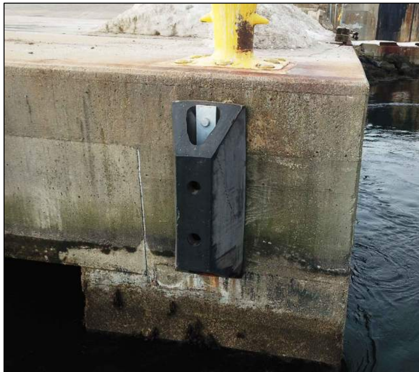
MAIN WHARF - FENDER SYSTEM LOOKING SOUTHWEST
