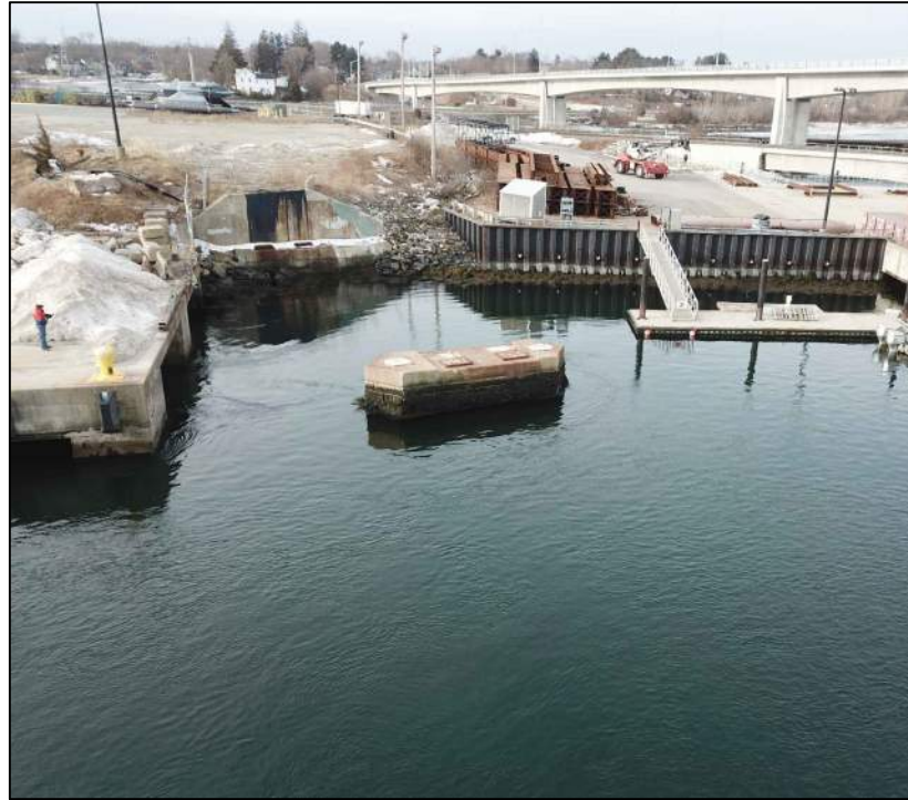
NORTH WHARF EXTENSION LOCATION LOOKING SOUTHWEST (C1)
