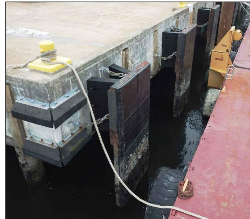
BARGE WHARF - FENDER SYSTEM LOOKING SOUTH
