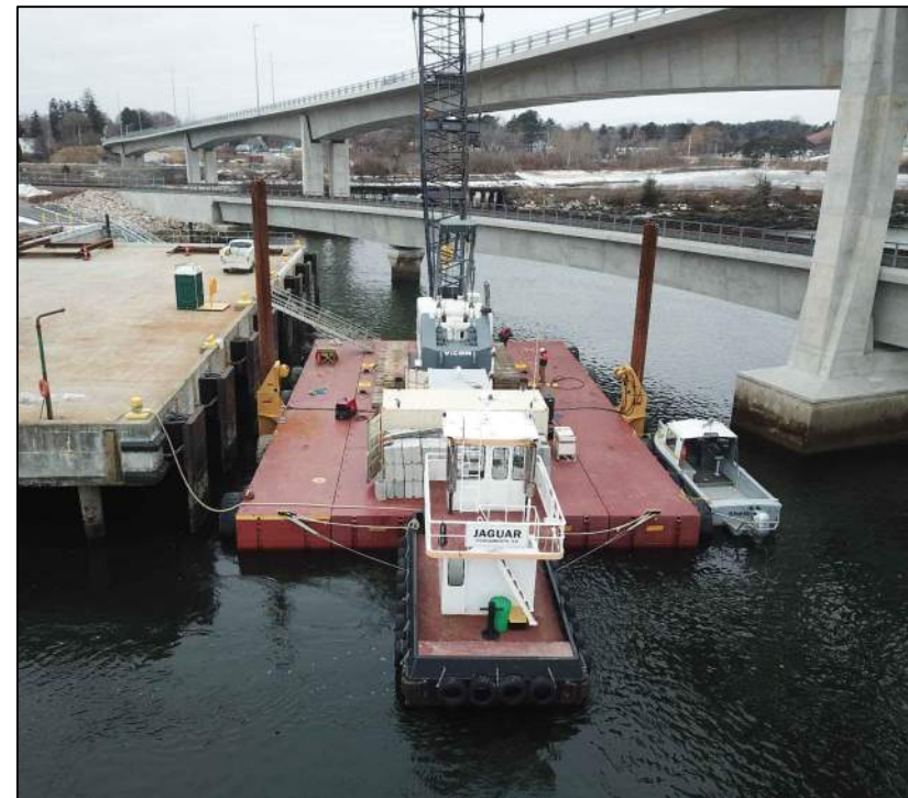
FLOATING DOCK - NEW LOCATION LOOKING SOUTHWEST (A4)
