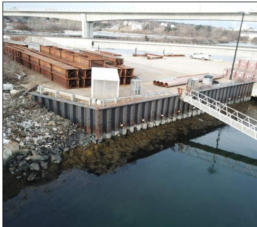
BARGE WHARF BULKHEAD LOOKING WEST (A1)
