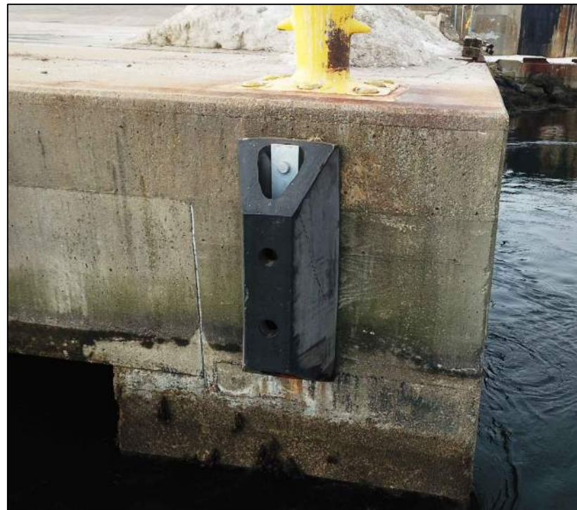
MAIN WHARF - FENDER SYSTEM LOOKING SOUTHWEST
