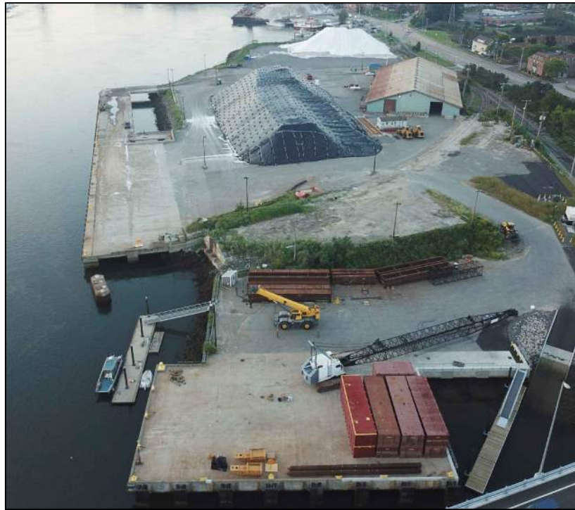
OVERALL SITE LOOKING SOUTHEAST
