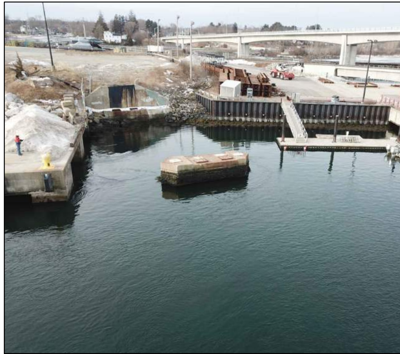
NORTH WHARF EXTENSION LOCATION LOOKING SOUTHWEST (C1)
