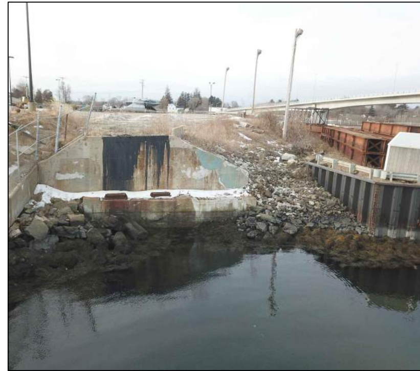
BRIDGE ABUTMENT 13 LOOKING SOUTHWEST (C4)
