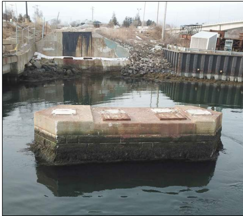
BRIDGE PIER 14 LOOKING SOUTHWEST (C3)
