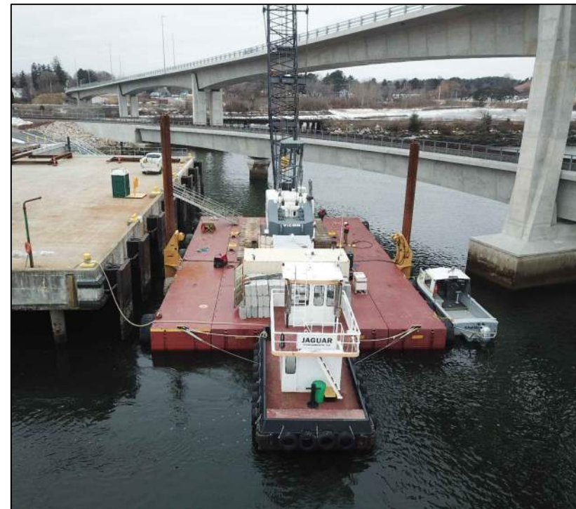
FLOATING DOCK - NEW LOCATION LOOKING SOUTHWEST (A4)
