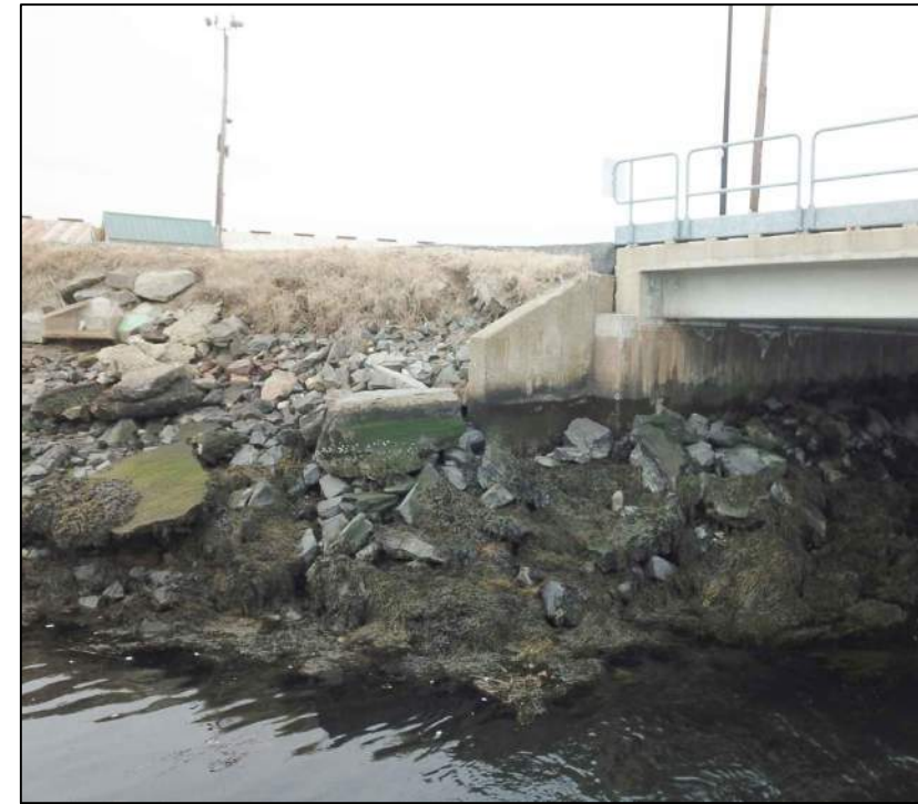
MAIN WHARF - BRIDGE ABUTMENT LOOKING WEST
