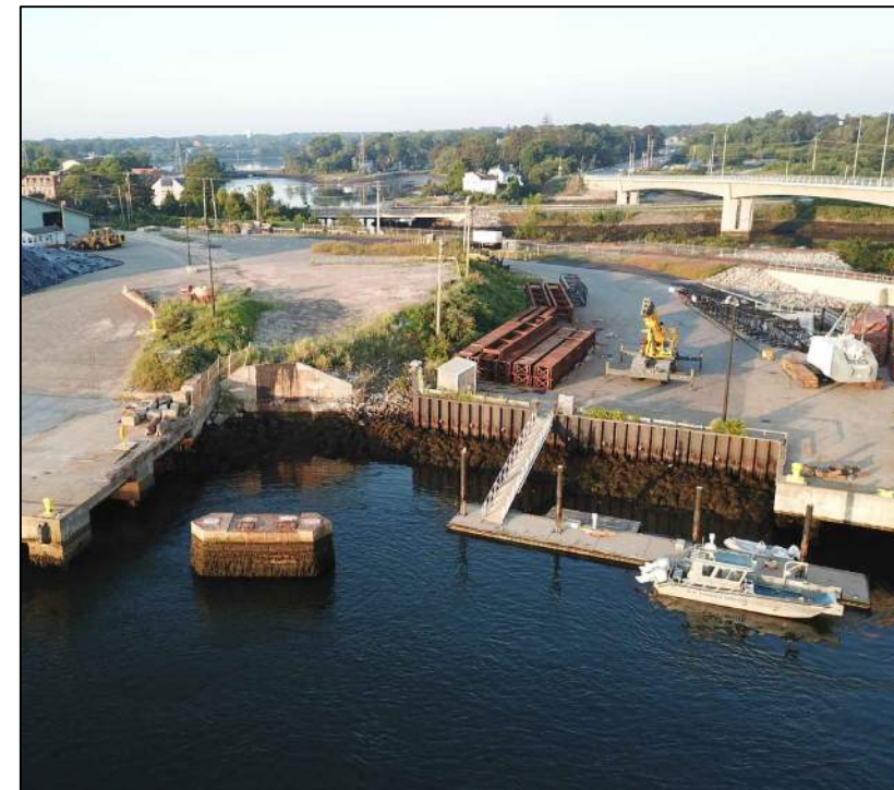
NORTH WHARF EXTENSION LOCATION LOOKING SOUTH
