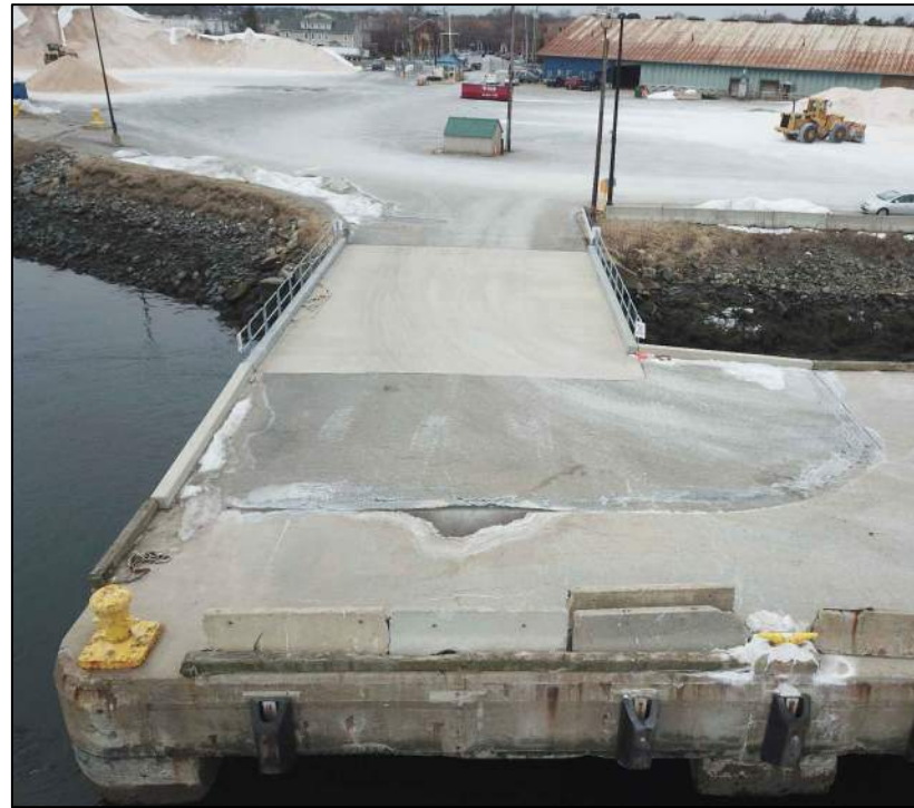
MAIN WHARF - SOUTH ACCESS BRIDGE LOOKING SOUTHWEST
