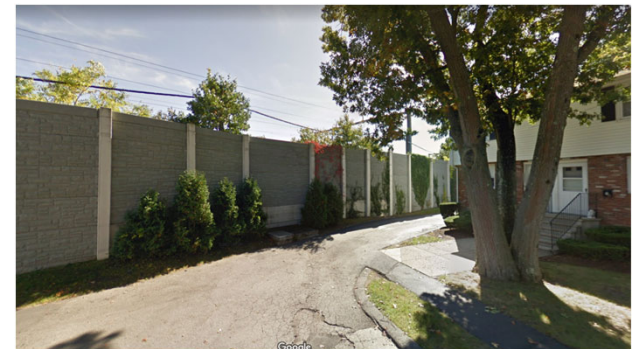
Typical noise mitigation wall adjacent to Readville rail yard
