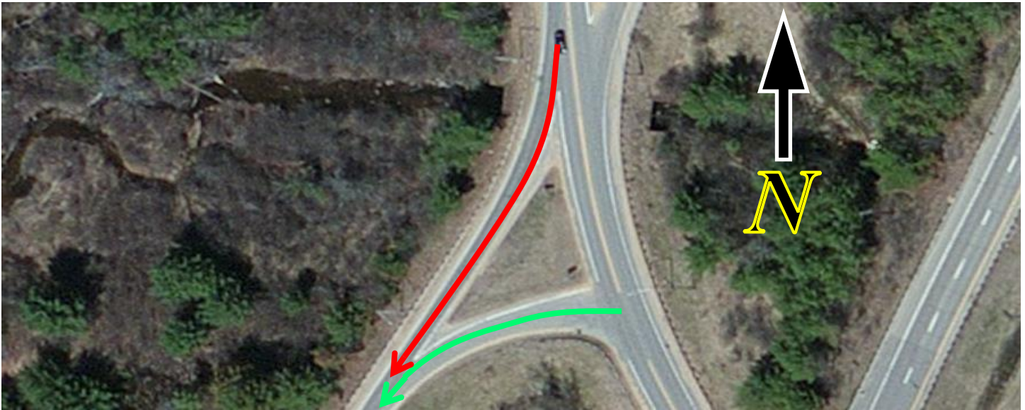
Ramp and slip ramp entering I-93 southbound from NH 132 in Northfield (Exit 19). The slip ramp (marked in red) can only be accessed while traveling south on NH 132; the primary ramp (marked in green) can be accessed from either direction. The slip ramp terminates when it meets the primary ramp. Note the island created between the primary ramp, the slip ramp, and the diverging route (NH 132).
