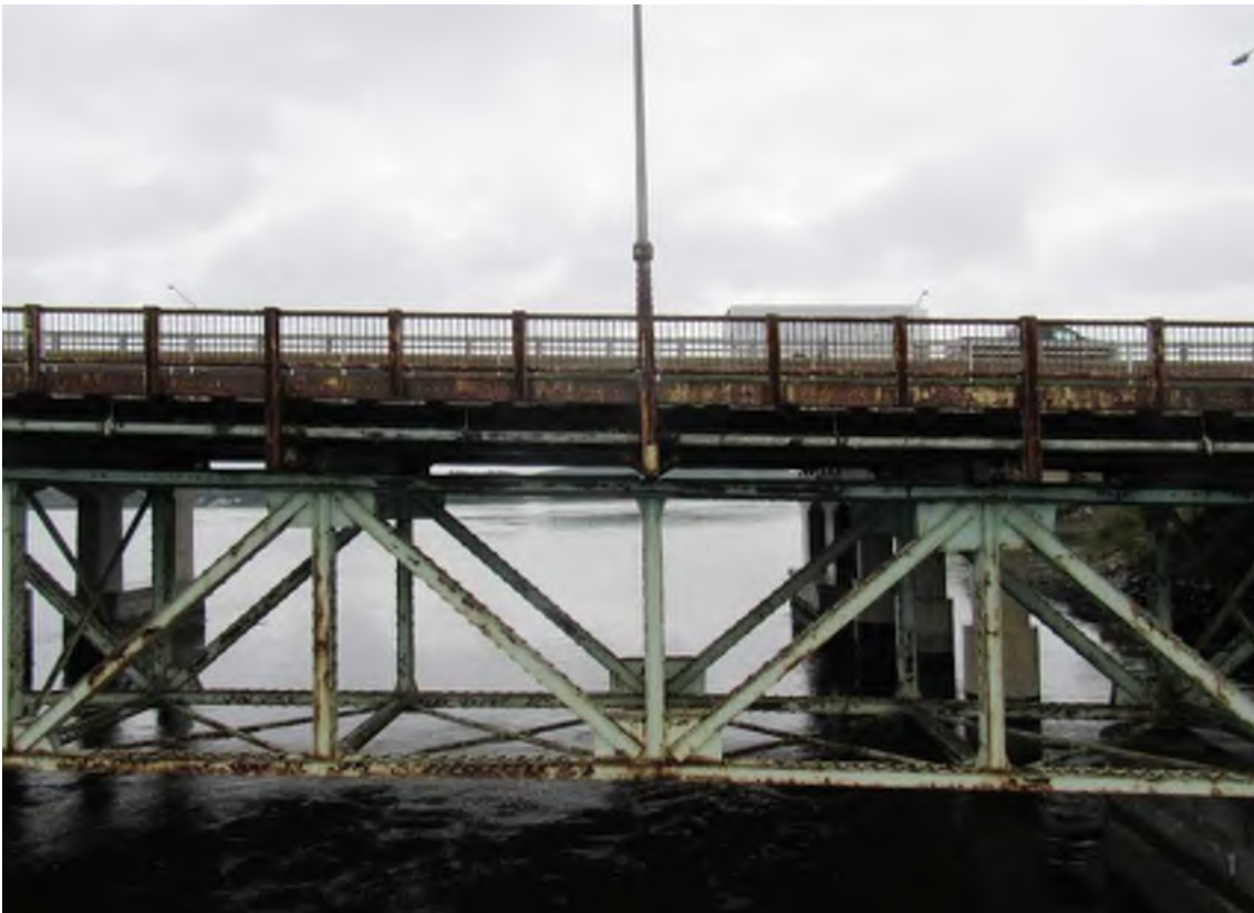
Photo 10: View east of the General Sullivan Bridge superstructure.
