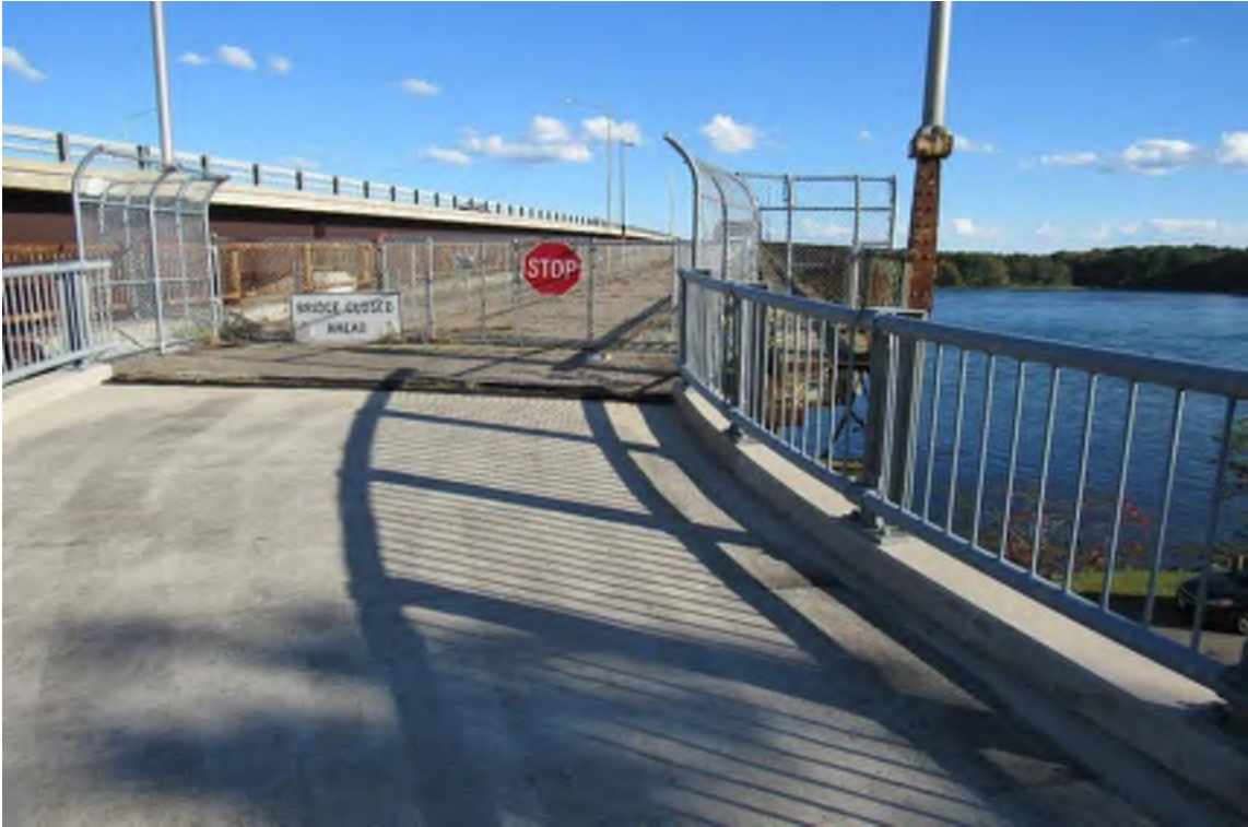
Photo 7: View north of the approach slab on the Dover side of the General Sullivan Bridge.
