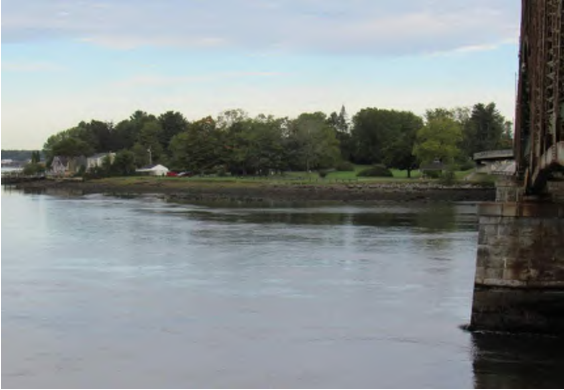
Photo 15: View north of Hilton Park and the Dover shoreline.
