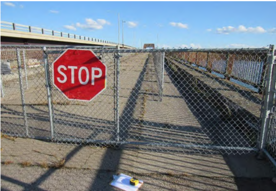
Photo 8: View north along the General Sullivan Bridge. The bridge has been closed since 2018.
