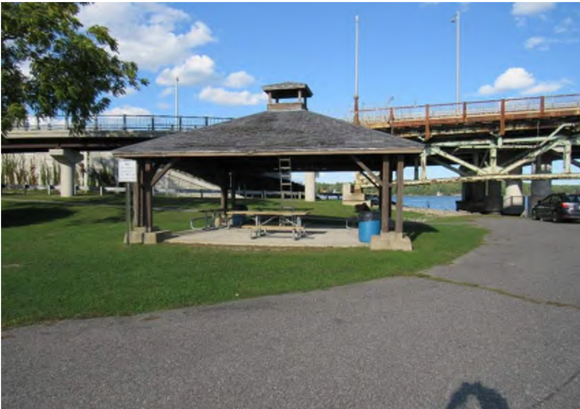
Photo 4: View west of the gazebo within Hilton Park that will be removed and replaced to provide a construction staging area for materials and equipment.
