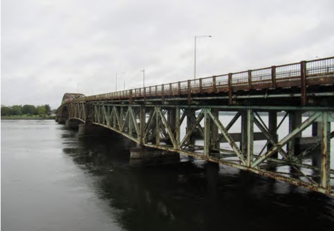
Photo 9: View north of the General Sullivan Bridge superstructure from Newington.
