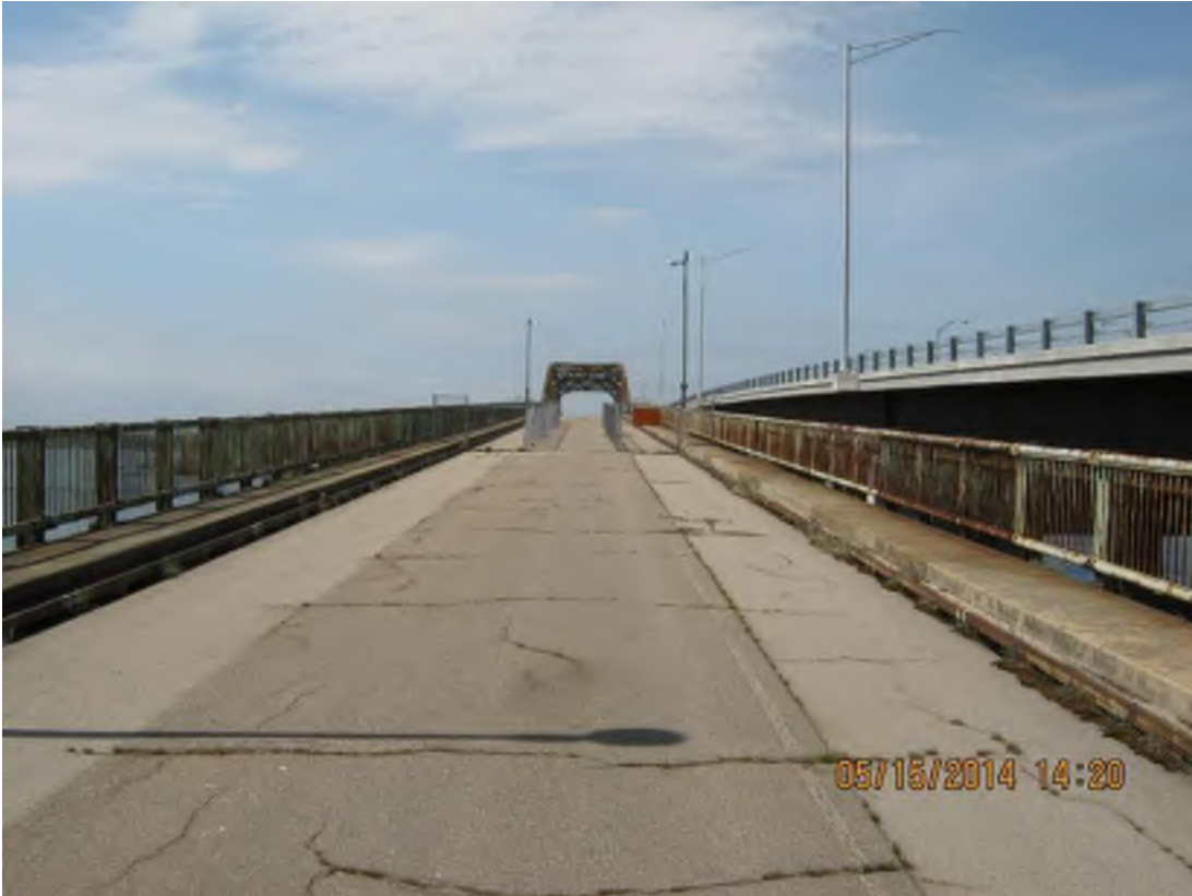
Photo 24: View north of the GSB along Newington approach.
