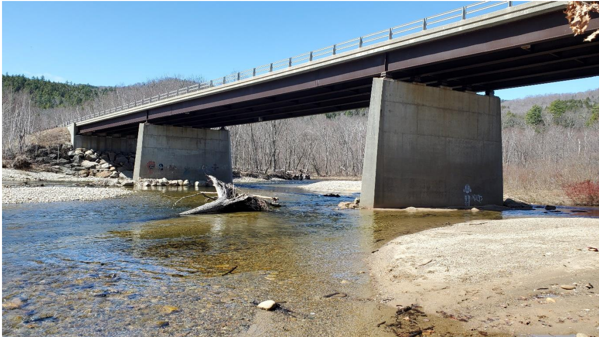
Figure 1. View of Bridge No. 195/093 with the Pemigewasset River flowing underneath (looking west). Pier I is on the left-hand side of the photo. Pier II is located on the right.
