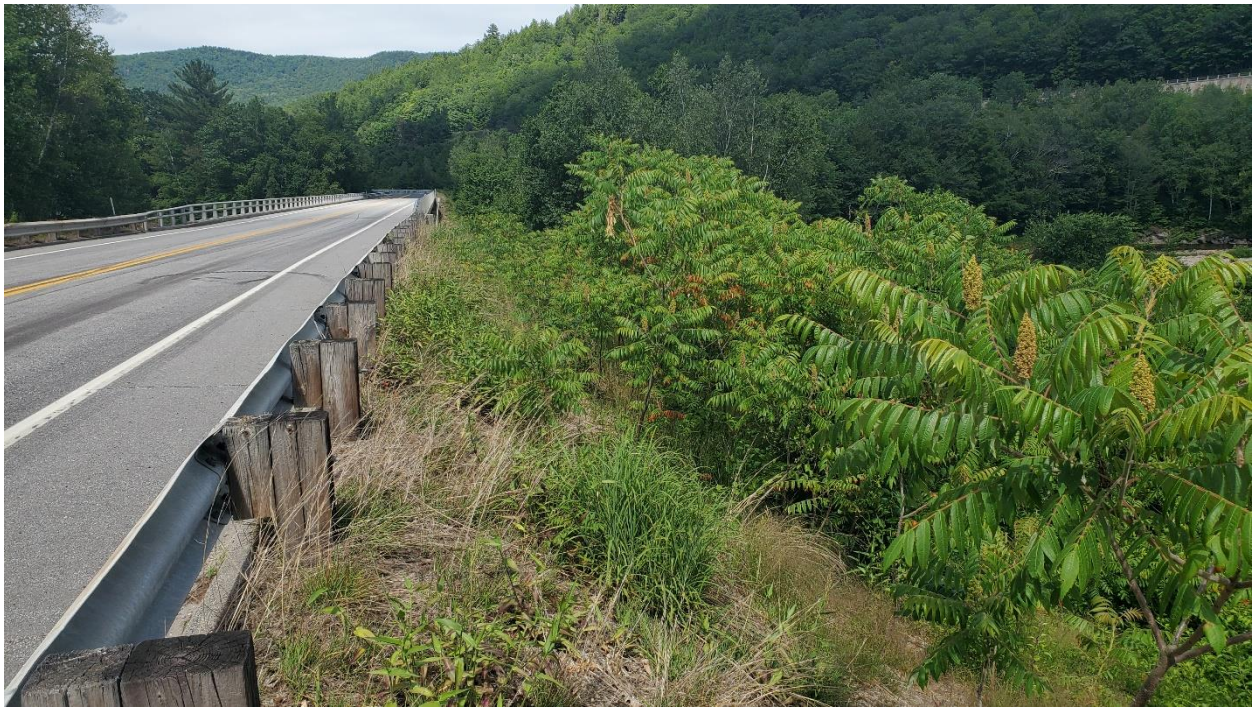
Figure 4. View of Route 175 (left side of photo) and slope where the temporary access road will be constructed to reach Pier 1 (looking northeast toward the bridge).
