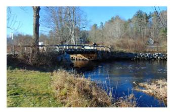
The existing bridge is a single span structure, originally constructed in 1850. In 1991 a concrete cap was installed on the existing stone abutments and the structure and decking were replaced. The existing structure consists of a wood deck, with associated wood timber curb, wood guardrail posts and steel girders, set on stone abutments. The structure is a single lane bridge, with a curb-to-curb travel lane width of approximately 12.3-feet.
