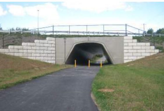
I-395 over Webster Avenue Pedestrian Tunnel
