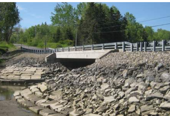
Mill Bridge over Mill Creek
