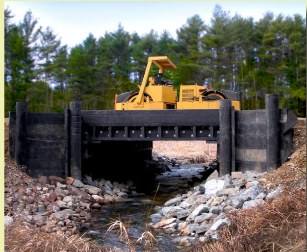
Birch Hill Road Culvert Replacement York, Maine
