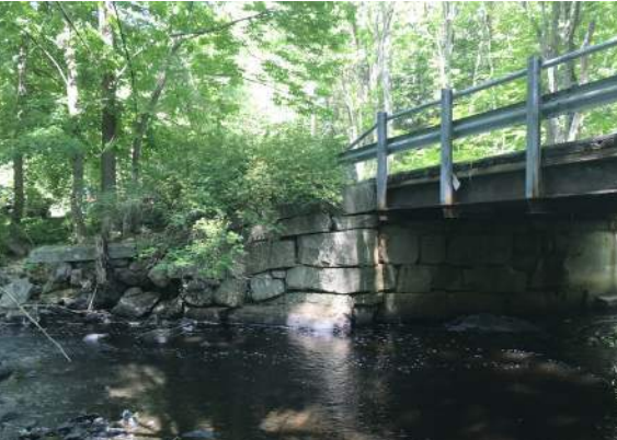
Staples Bridge over Great Works River
