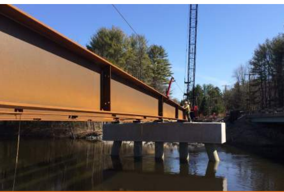
Covered Bridge over Little Androscoggin River
