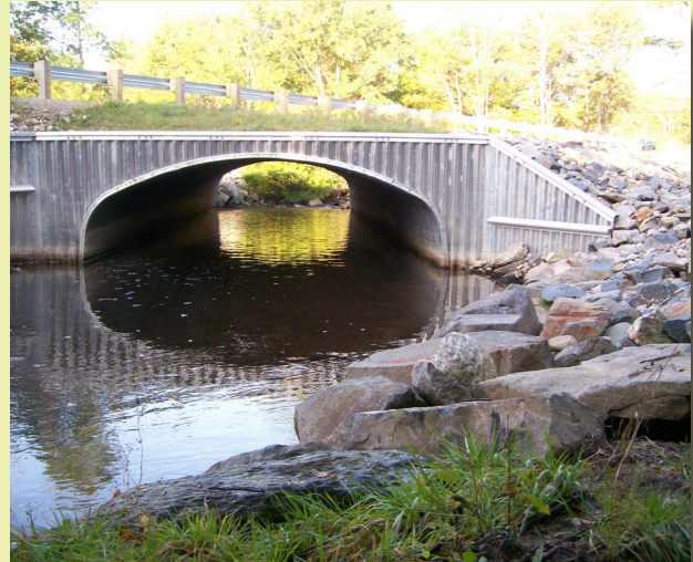
Chesley Hill Road Bridge After Reconstruction Rochester, New Hampshire
