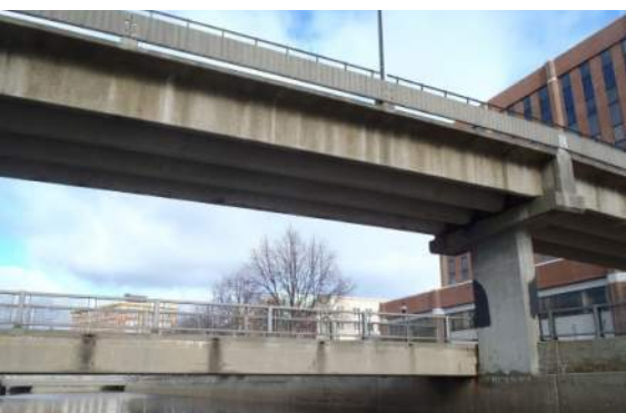
Kenduskeag Stream "At Grade" Pedestrian Bridge
