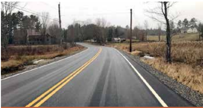
NH Route 113 after construction of twin 15-Inch RCP culverts with headwalls.
