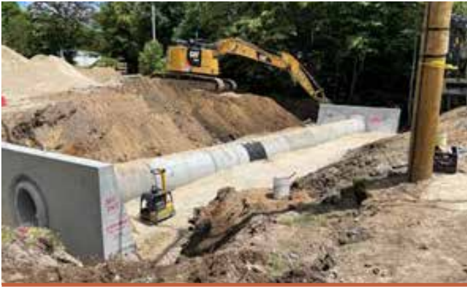
The district replaced a 42-inch RCP under NH Route 108 in Dover. The work required a four-day road closure with utility coordination.
