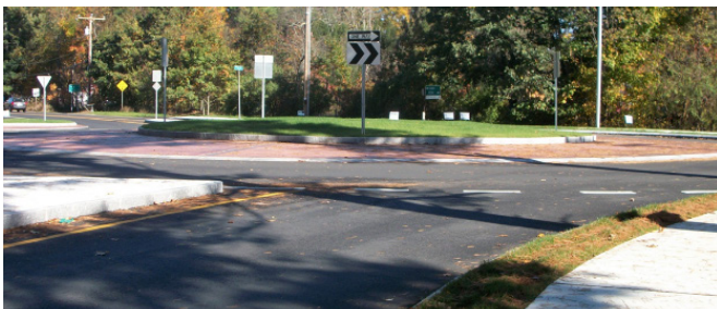
The Maple Ave Roundabout project in Keene was funded by a HSIP Program grant and needed to be fast-tracked to meet HSIP Funding deadlines. CHA completed the design and permitting in just over three months.
