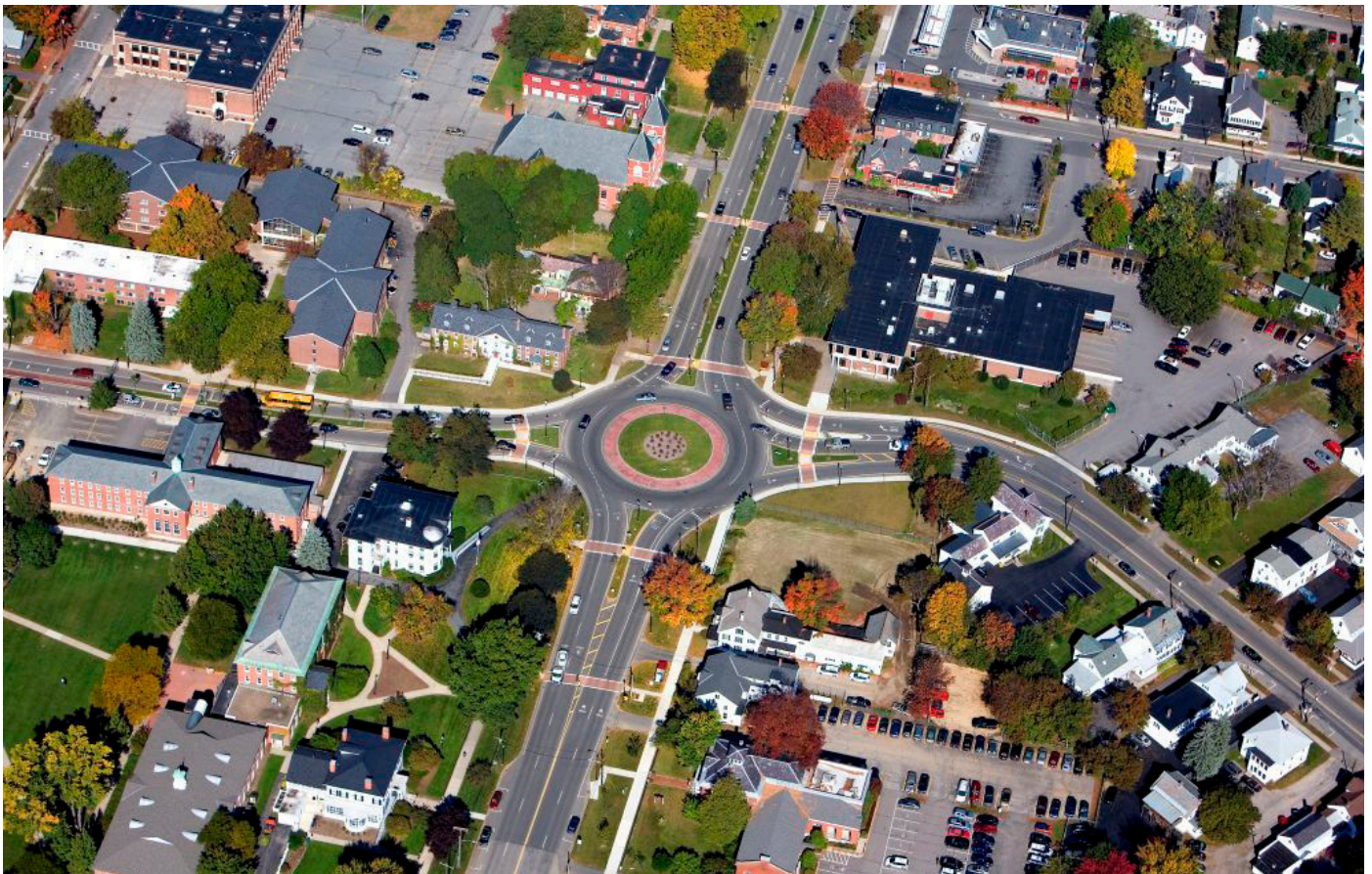
Winchester, Main, and Marlboro Street Intersection Preliminary and Final Design Improvements, Keene, NH
