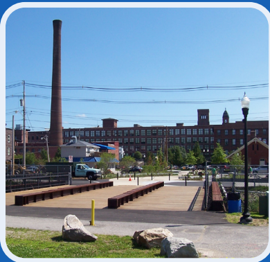
Simard-Payne Pedestrian Bridge Lewiston, ME
