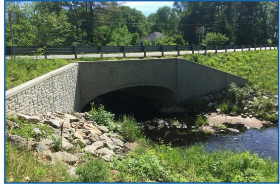
**Buried structures provide an economical, environmentally friendly, and low maintenance solution for many small bridges.**
