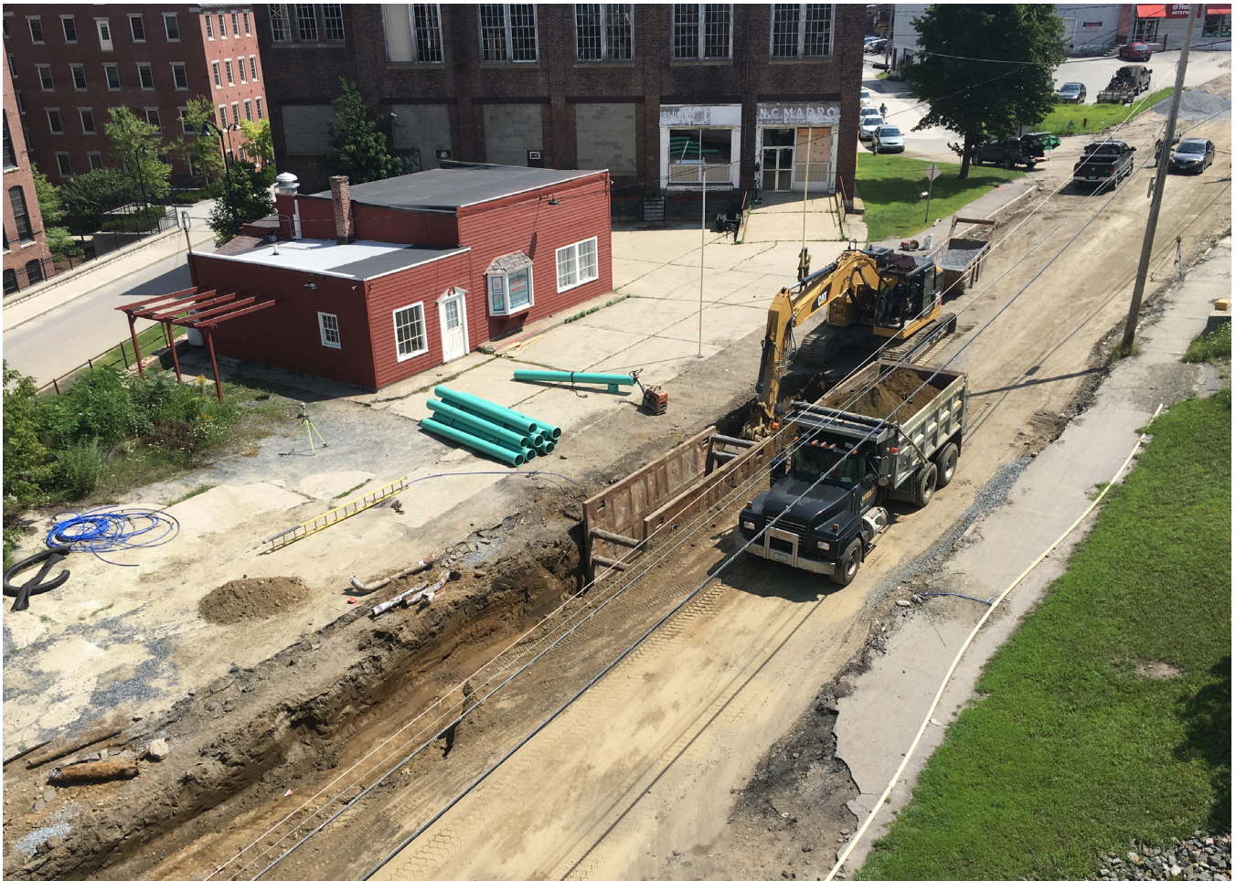
Pleasant Street Reconstruction, Claremont
