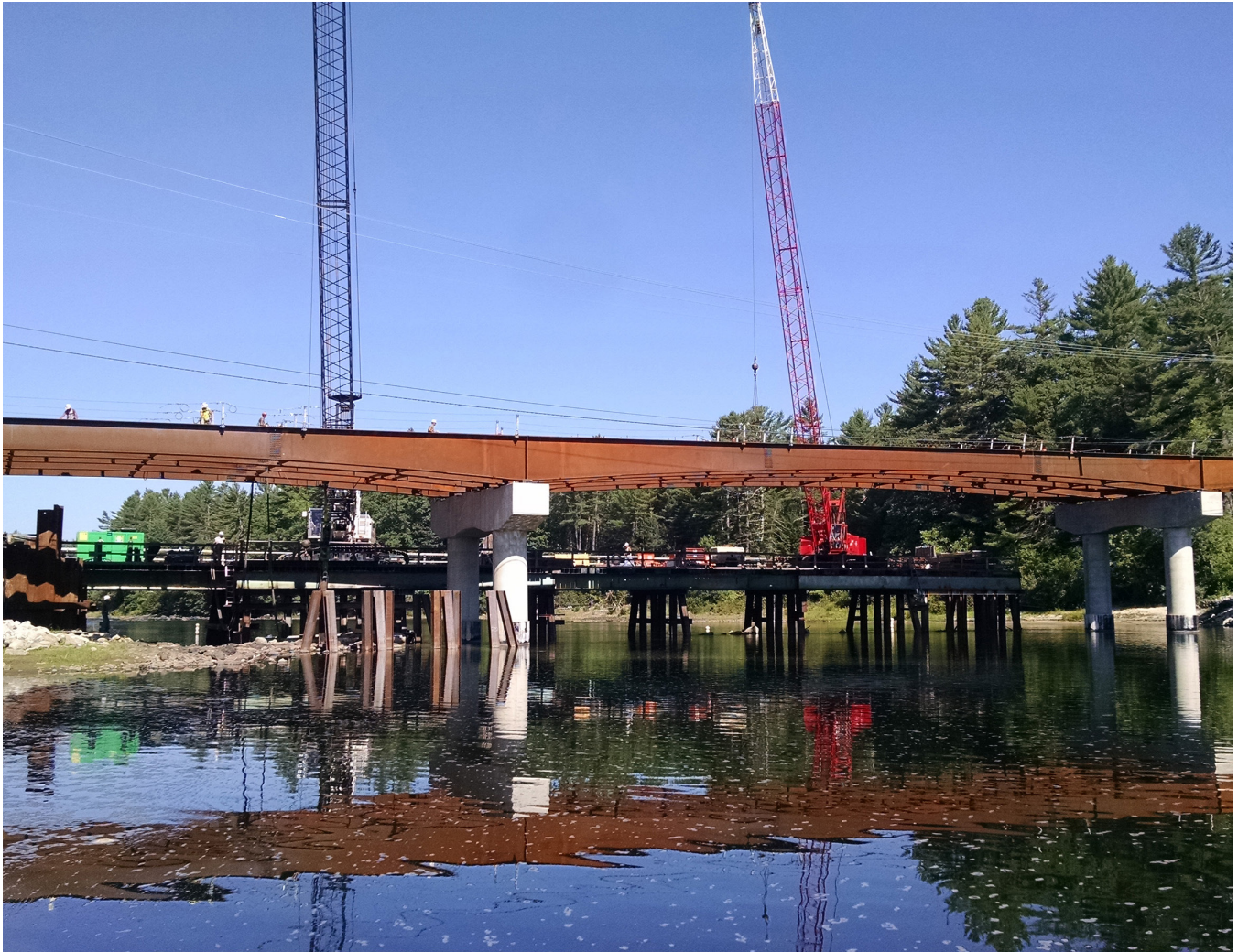
Sewalls Falls Bridge Construction, Concord
