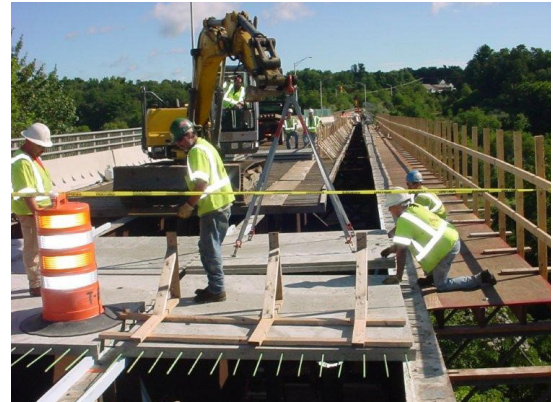
Kelley Street Bridge Deck Construction, Manchester
