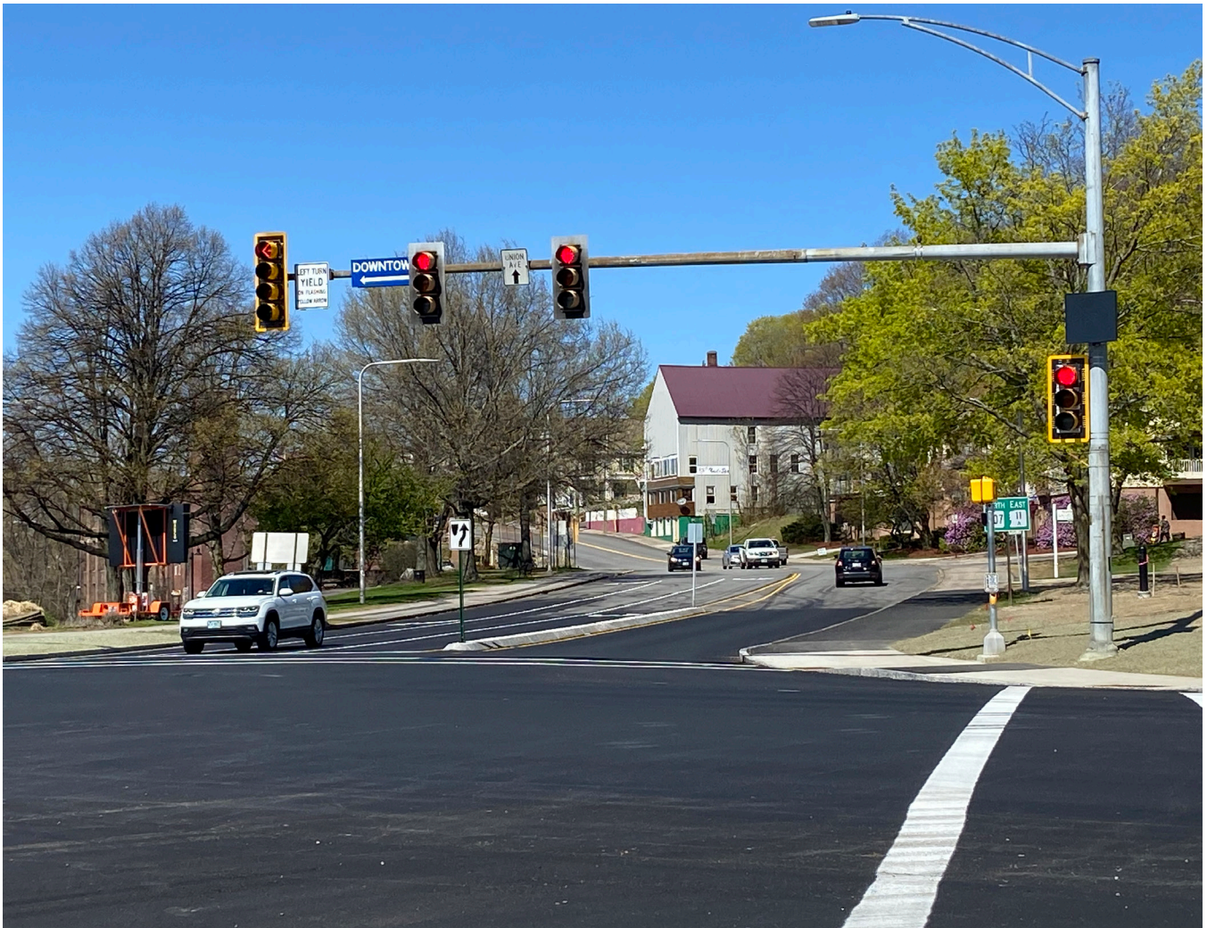
Court Street Rehabilitation, Laconia
