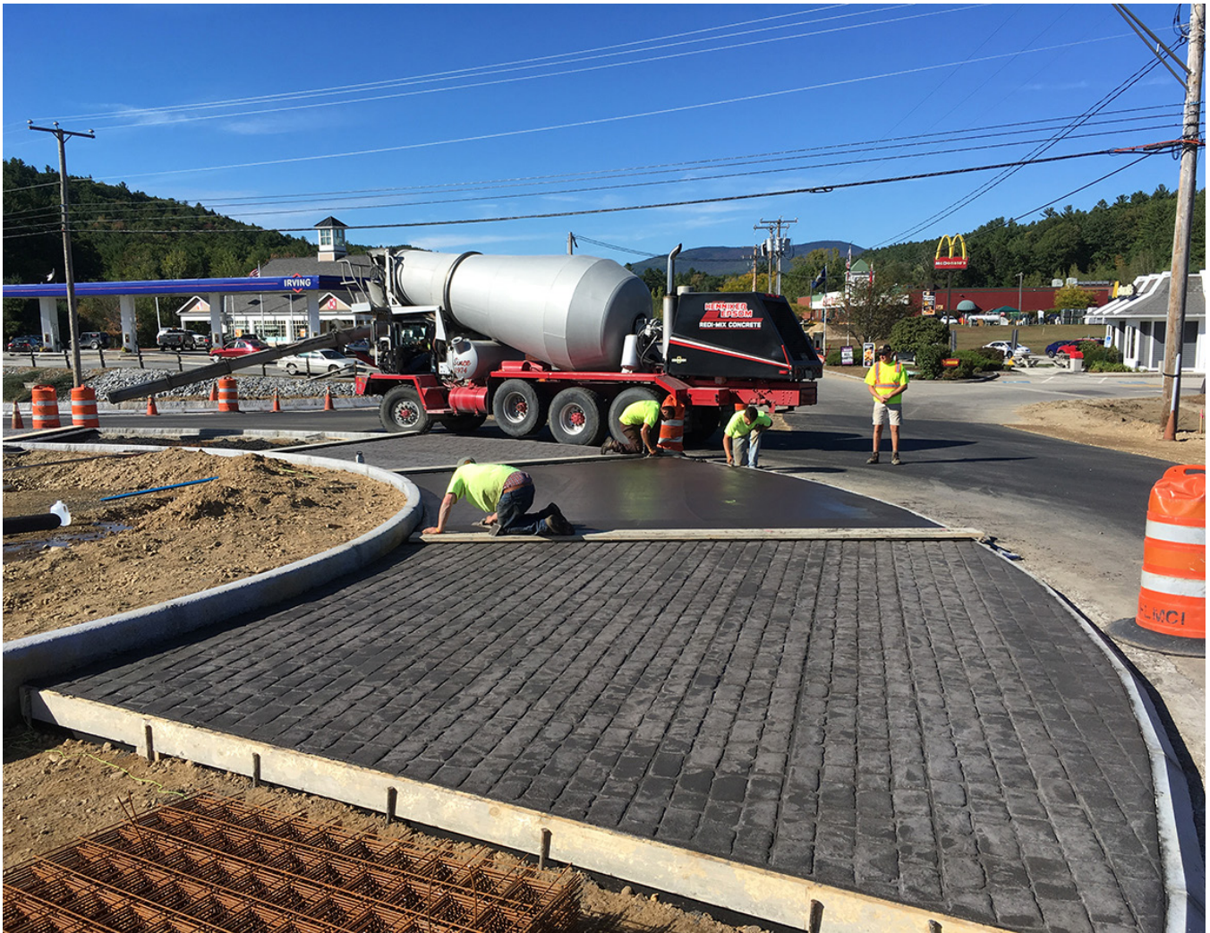
Route 103 Traffic Calming and Roundabout, Warner
